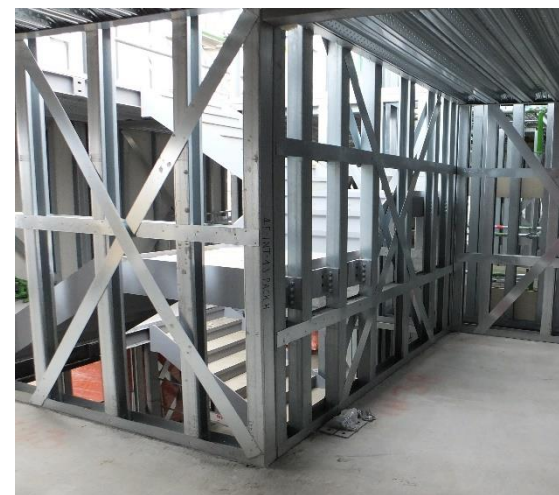
Load bearing framing
