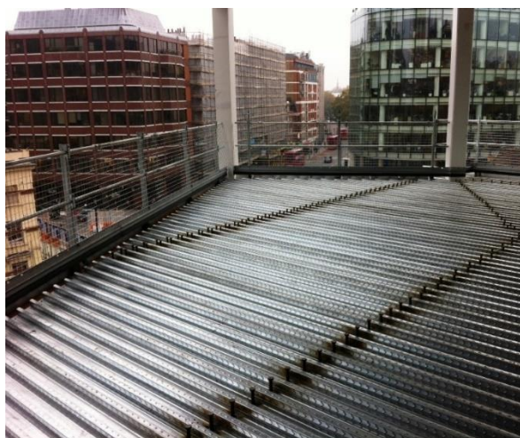
Metal decking and studs
