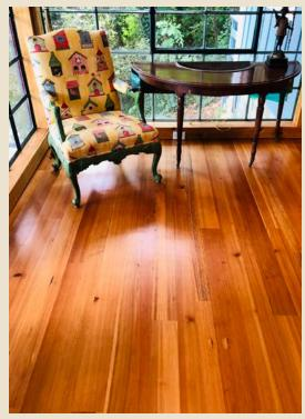
Our **VERTICAL GRAIN HEART PINE** has long been cherished as one of the most stable old-growth woods. It is noted for its deep amber color and tight, straight grain lines. The antique lumber is sawn perpendicular to the growth rings to achieve this special effect, producing a very durable wear surface with few knots (often called quartersawn or rift-sawn). This floor is our premium product with heart content above 90%. This beautiful wood floor will grow richer and darker each year.
