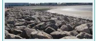
Cost per m (£): 1000 Aesthetics: Natural rock Life span: 25 years Benefits: Still allows some natural processes to occur. Relatively quick construction. Issues: Can be undermined or moved by large waves. Requires some maintenance.
