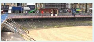
Cost per m (£): 6000 Aesthetics: Concrete Life span: 100 years Benefits: Prevents flooding and erosion. Issues: Long construction process.
