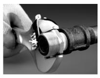
Step 6 Attach flange nut to the installed HOME-FLEX® fitting
