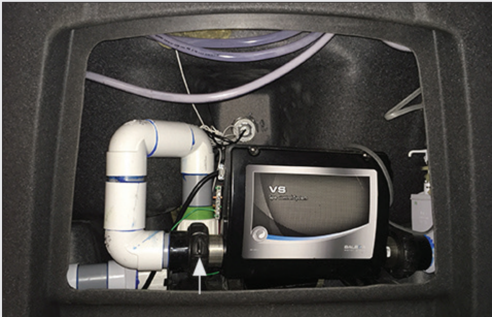
FIGURE 1.9 : HEATER UNION; LOOSEN UP TO BLEED AIR
