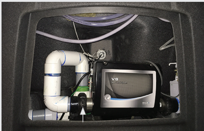
FIGURE 1.9a : HEATER UNION; LOOSEN UP TO BLEED AIR
