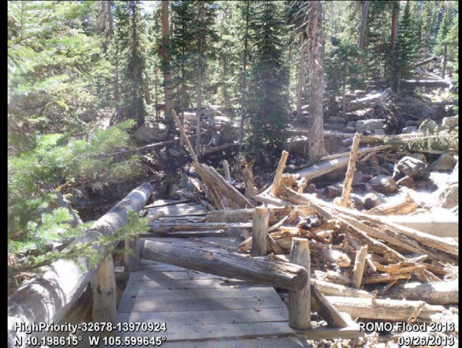
Bridge damage on the Ouzel Falls Trail
