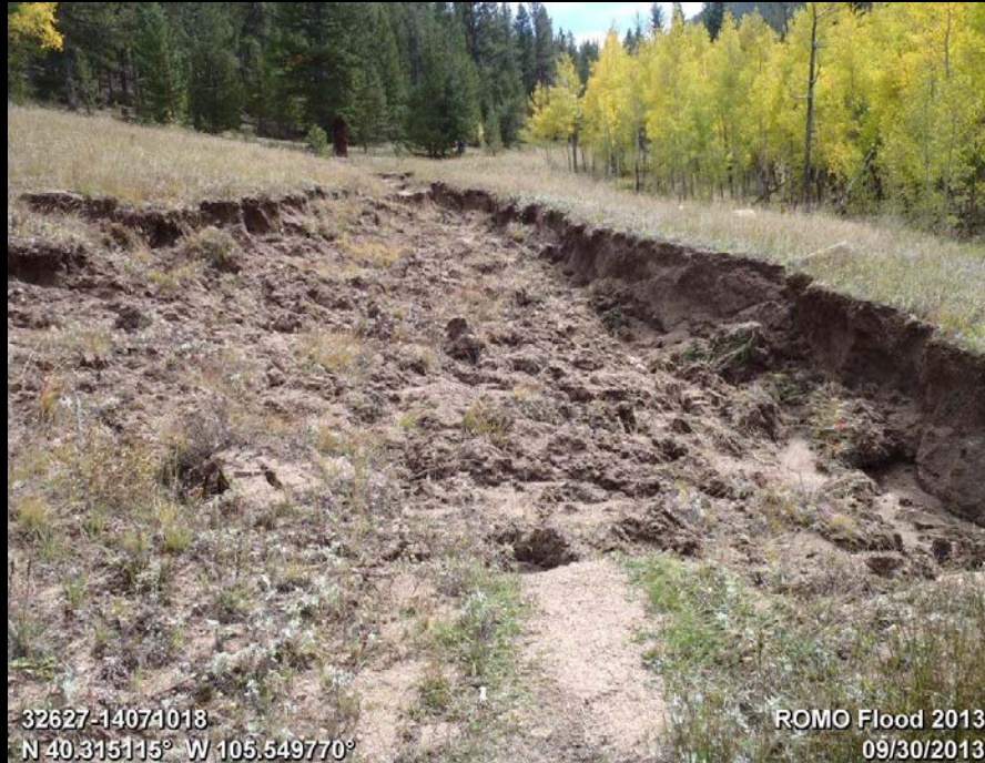
Collapsed Tread on the Aspen Brook Trail
