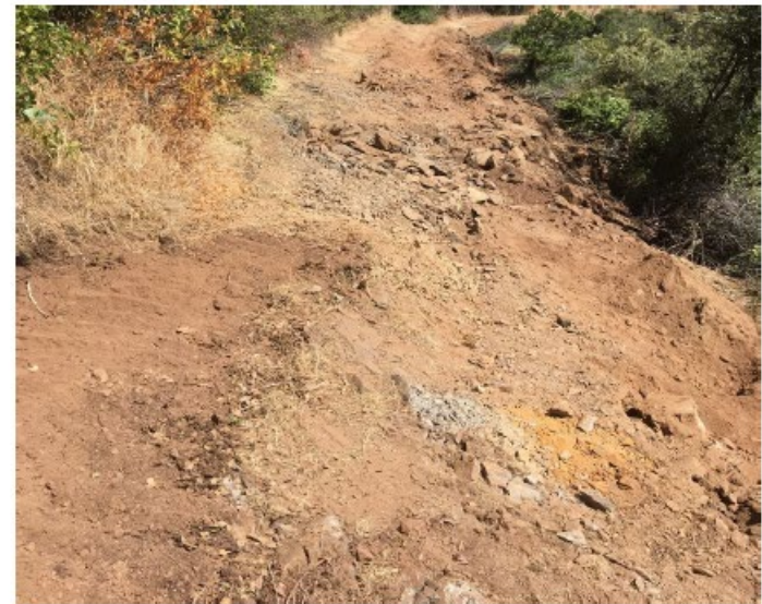
View looking north along the trail at the fall site
