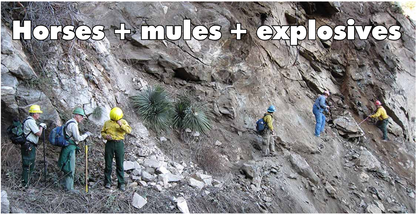
The bulging cliff overhang that needed to be blasted to prepare a shelf for trail construction
