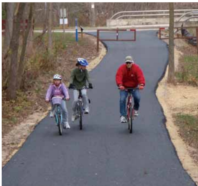
Porous asphalt was used to surface Pheasant Branch Conservancy Trails in Middleton, Wisconsin
