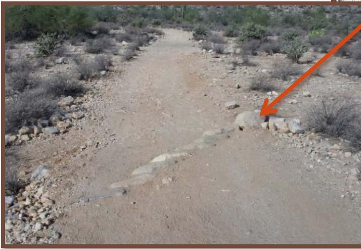
A finished waterbar has an appearance similar to a grade dip. Use fill material to create an embankment against the downgrade side of the waterbar to act as a ramp. A smaller embankment is compacted against the upgrade side to serve as a shorter ramp and to guide water into the drain spillway.
