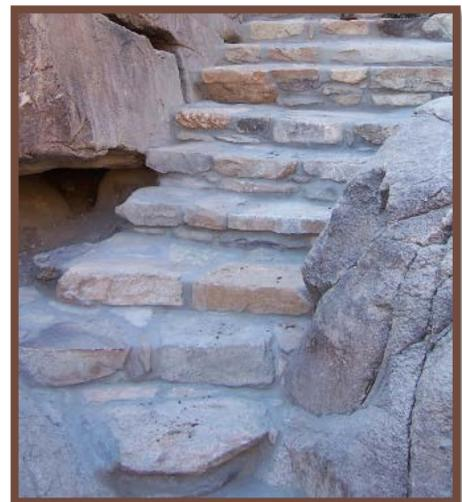
in shape; use tools to shape the rocks if necessary. Each rock must be large and heavy enough to be stable and meet rise and run requirements. Excavate a terrace, hand place each rock, and compact soil around rocks to ensure stability. Utilize concrete block to level the ground and provide additional support for the steps.
