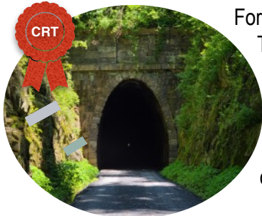
West Portal Blue Ridge Tunnel, VA Photo Credit: Nelson County
