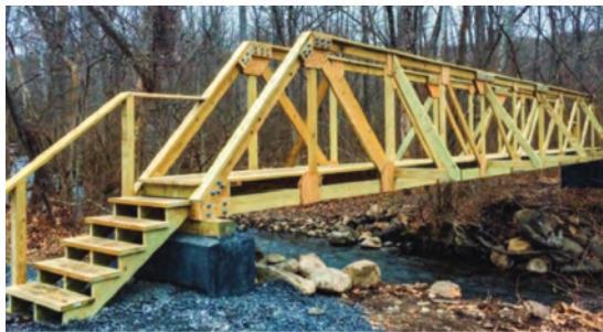
Highlands Trail bridge connects trails to 4 States, NJ Photo Credit: Kylie Yang
