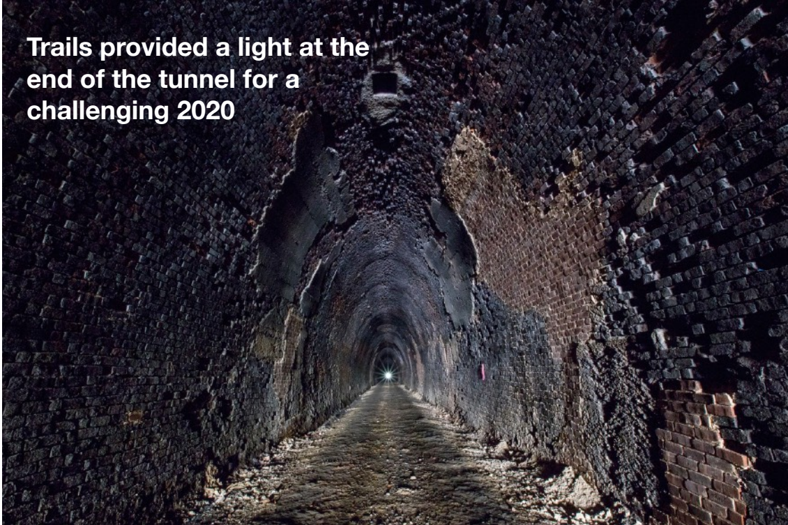
West looking east tunnel interior of the Blue Ridge Tunnel Rehabilitation & Trail Project, VA Photo Credit: Nelson County
