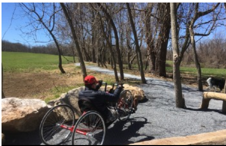
Hardened surface trail improves access, DE Photo Credit: David Bartoo DNREC
