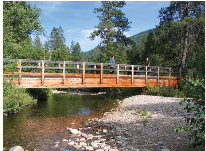
Figure 3—A glued-laminated (glulam) deck girder trail bridge.
