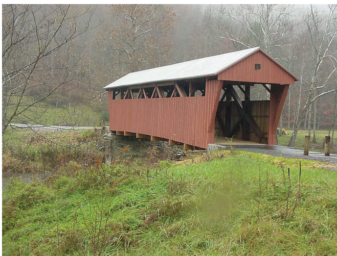
Figure 8—Many old covered bridges are being converted into pedestrian bridges.
