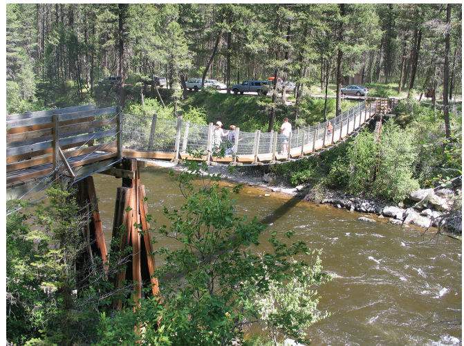
Figure 7—A deck cable bridge supported by two main cables on timber towers.
