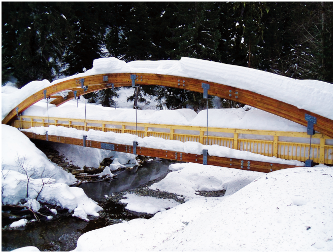
Figure 10—Trail bridges should be designed for snow loads.
