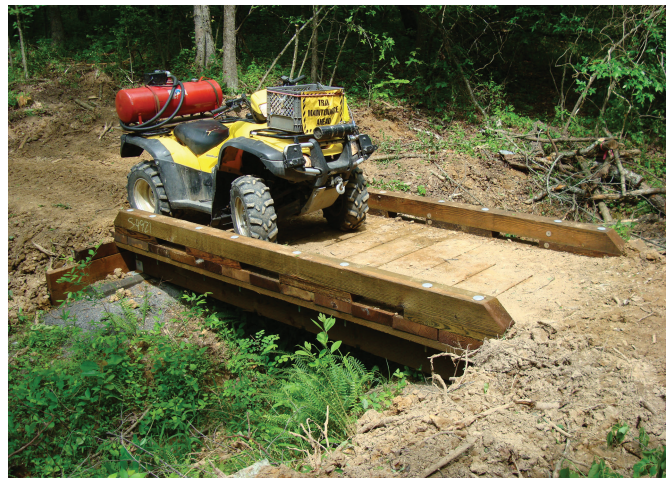
Figure 9—A single-unit timber bridge designed to accommodate all-terrain vehicles, bicycles, and hikers.
