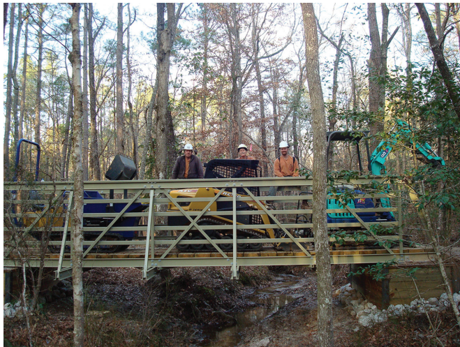
Figure 11 – Trail bridges should be designed to support applicable trail maintenance equipment.
