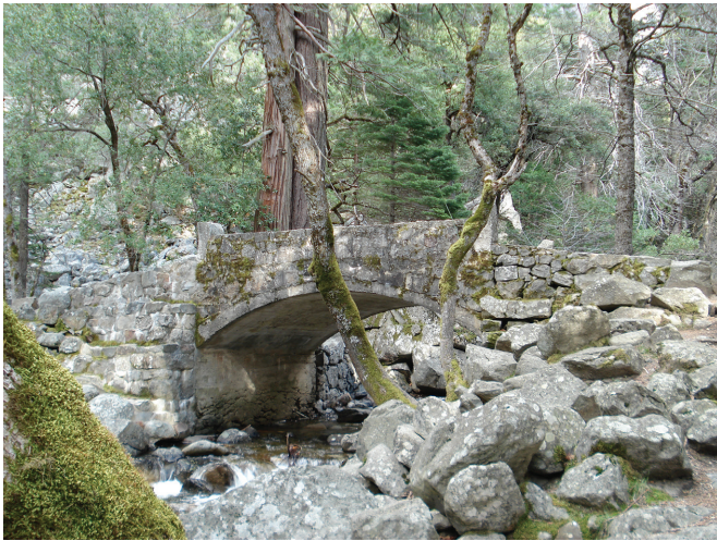
Figure 6—This masonry arch trail bridge was originally constructed for vehicle traffic.
