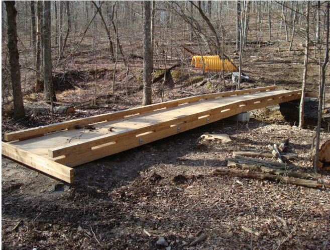
Figure 4—A single-unit bridge with two timber slabs.
