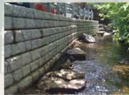
TOE ROCK WALL PROTECTION
