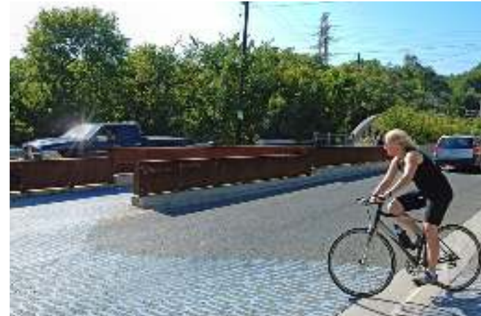
Creative use of pavement markings to indicate the path of travel through a refuge island at the intersection of the Lower Don Trail and Pottery Road
