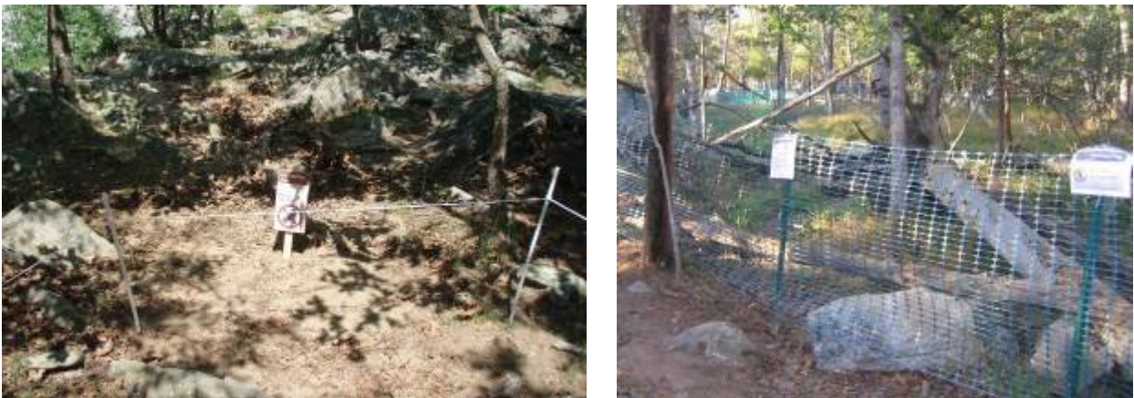
Figure 2. Low symbolic post and rope fencing (left) and high fencing designed to physically obstruct access (right).
