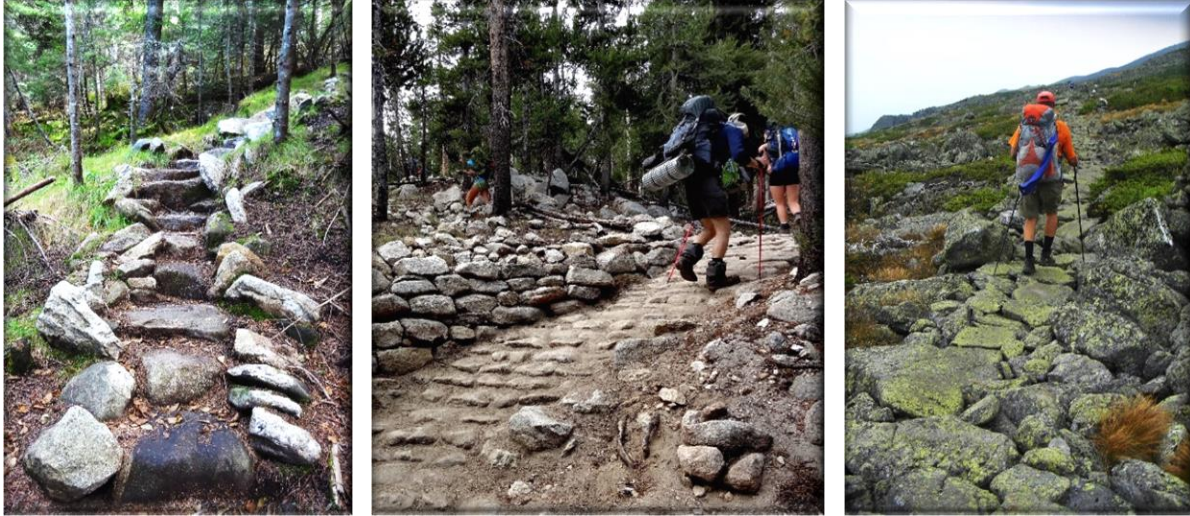
Figure 29. Tread construction with stone steps or stone armoring of trail treads can help minimize soil loss in steep terrain.
