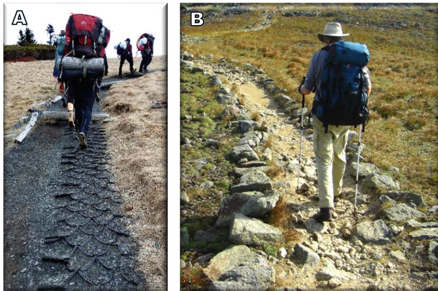
Figure 30. Cellular geotextile products (A) can retain soils within their 3-D cells but fill material placed on top will erode or displace downhill, exposing it to traffic and UV-radiation that breaks down the plastic. Its efficacy is higher in flat terrain and wet soils. Rock borders and scree walls (B) can be an effective practice for centering traffic and deterring off-trail travel.
