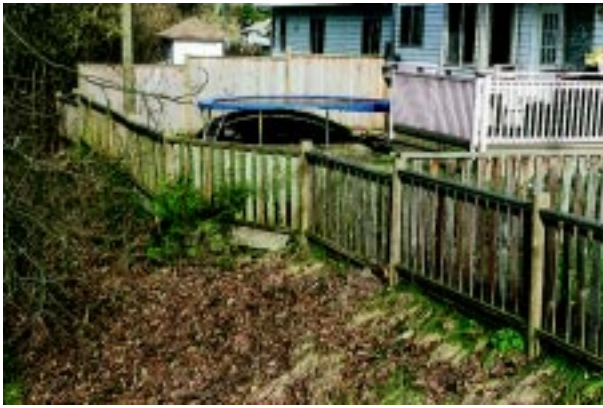
A rugged 6 ft. timber fence with vertical slats is aesthetically pleasing and has been successful in preventing trespass into a ravine and stream corridor
