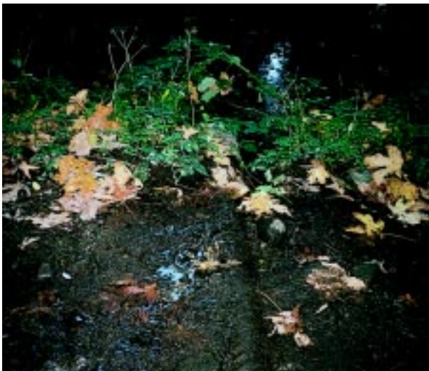
Poor cross drainage has led to erosion and has accelerated trail wear
