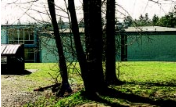
This large high school lacks barriers and invites students to congregate in a ravine adjacent to an ESA
