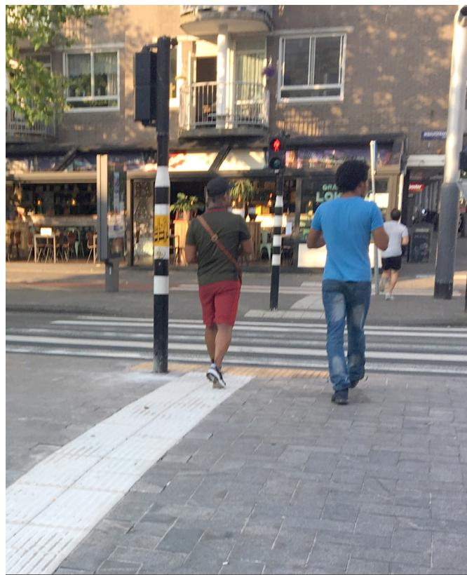
Figure 11: Example from the Netherlands of how directional indicators can be used to guide pedestrians to a crossing location. Note how the color of the indicator contrasts visually with the adjoining surface
