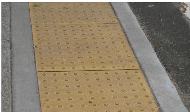
Figure 9: Example of a yellow detectable warning surface used at a shared use path crossing.
