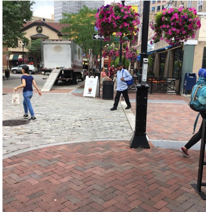
Figure 13: On this shared street, the cobbled surface of the shared zone is detectably different from the smooth bricks used in the comfort zone and crosswalks. The gray of the cobbled surface also contrasts visually from the red bricks. Note that cobbles should not be used in the pedestrian access route. SOURCE: Accessible Design for the Blind
