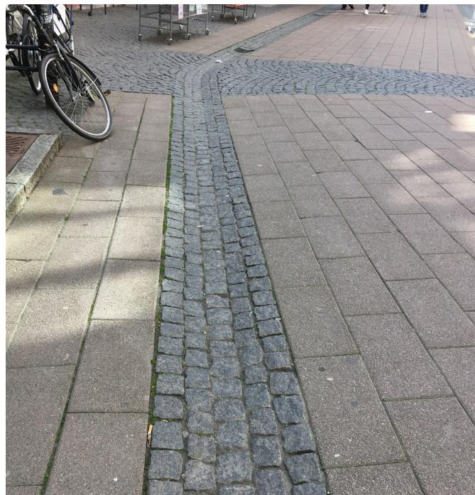
Figure 14: This shared street uses a valley gutter to indicate the edge of shared zone. The detectability of this valley gutter is enhanced because it is made of small granite cobbles. Note that cobbles should not be used in the pedestrian access route. SOURCE: Accessible Design for the Blind
