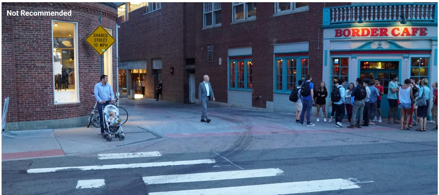
**Figure 20:** The design of this shared alley includes a detectable warning surface across the alley exit; however, the marked crosswalks are to the right and left of the alley exit.
