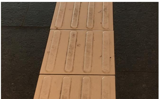
Figure 10: Example of a directional indicator.
