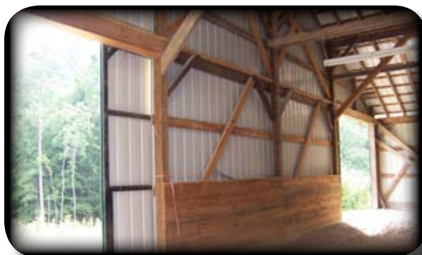
Double bank of stalls located in the center
