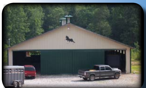
Front of building has double sliding doors.
