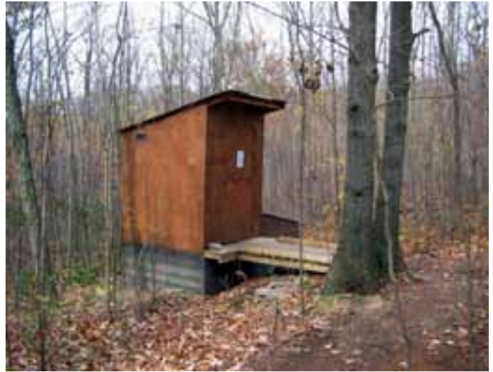
Composting Toilet along the Appalachian Trail ©Jeffery L. Marion
