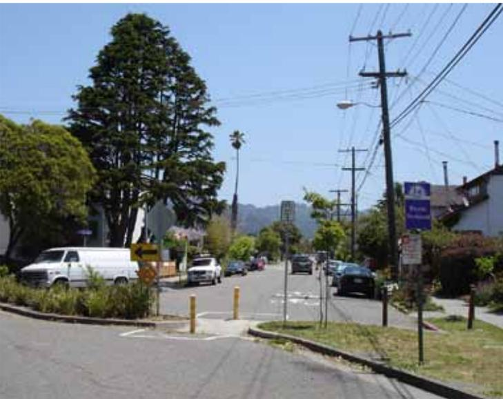
Street closures and diverters allow through bicycle traffic and reduce motor vehicle volumes and speeds.
