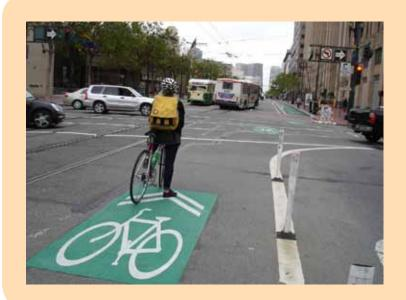
SFMTA has installed "green backed" sharrows through intersections on Market Street that are standard white sharrows on a green box that adds emphasis to the marking. The green backed sharrows assist bicyclists in positioning themselves correctly for the cycle track as it transitions to and from the curb in different segments.
