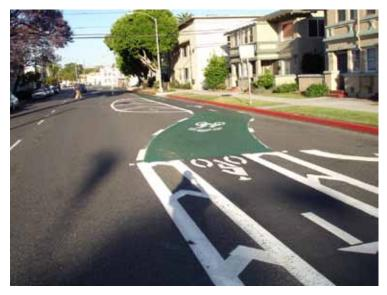
Above and below are two examples of through bike lanes indicating where bicyclists should shift over to allow motor vehicle left turns along the Long Beach cycle track.
