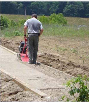
**Soil cement** is a mixture of pulverized native soil, Portland cement and water, rolled and compacted into very dense surface. It is cheaper than asphalt, but implementation of measures to allow adequate drainage is very important to prevent erosion and deterioration of the trail.
