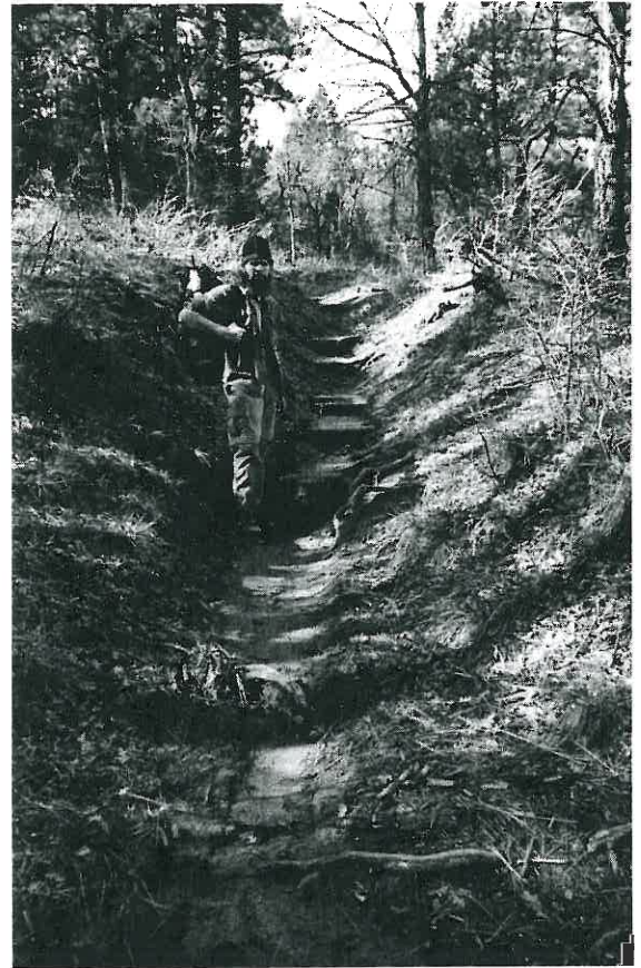
Fig. 13.2. It is impossible to drain water out of this entrenched trail in Zion National Park, USA, due to its low slope alignment angle. Re-routing is recommended to avoid the need for extensive tread work involving erosion control measures and steps on the existing alignment.
