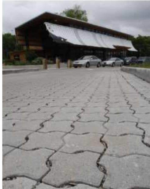
This shared street is an application of **design flexibility** that meets the needs of all users, while doubling as stormwater management, capturing the first inch of runoff during storm events and eliminating nuisance flooding. After completion, the project won the Tennessee Governor’s Environmental Stewardship Award for Excellence in Green Building as well as a Chattanooga Low Impact Development Excellence Award.
