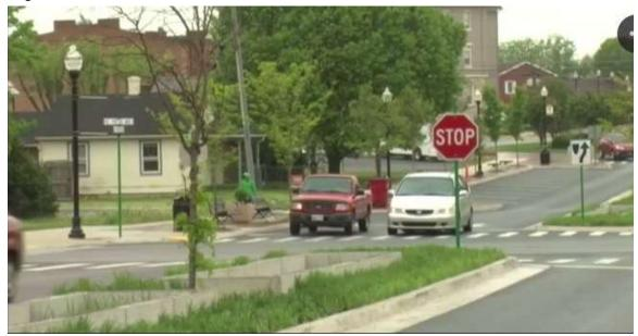
Median bioswales capture and filter stormwater runoff.
