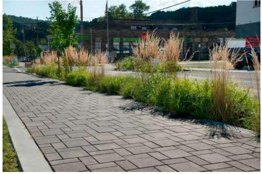
Permeable pavers and bioswales improve stormwater management.
