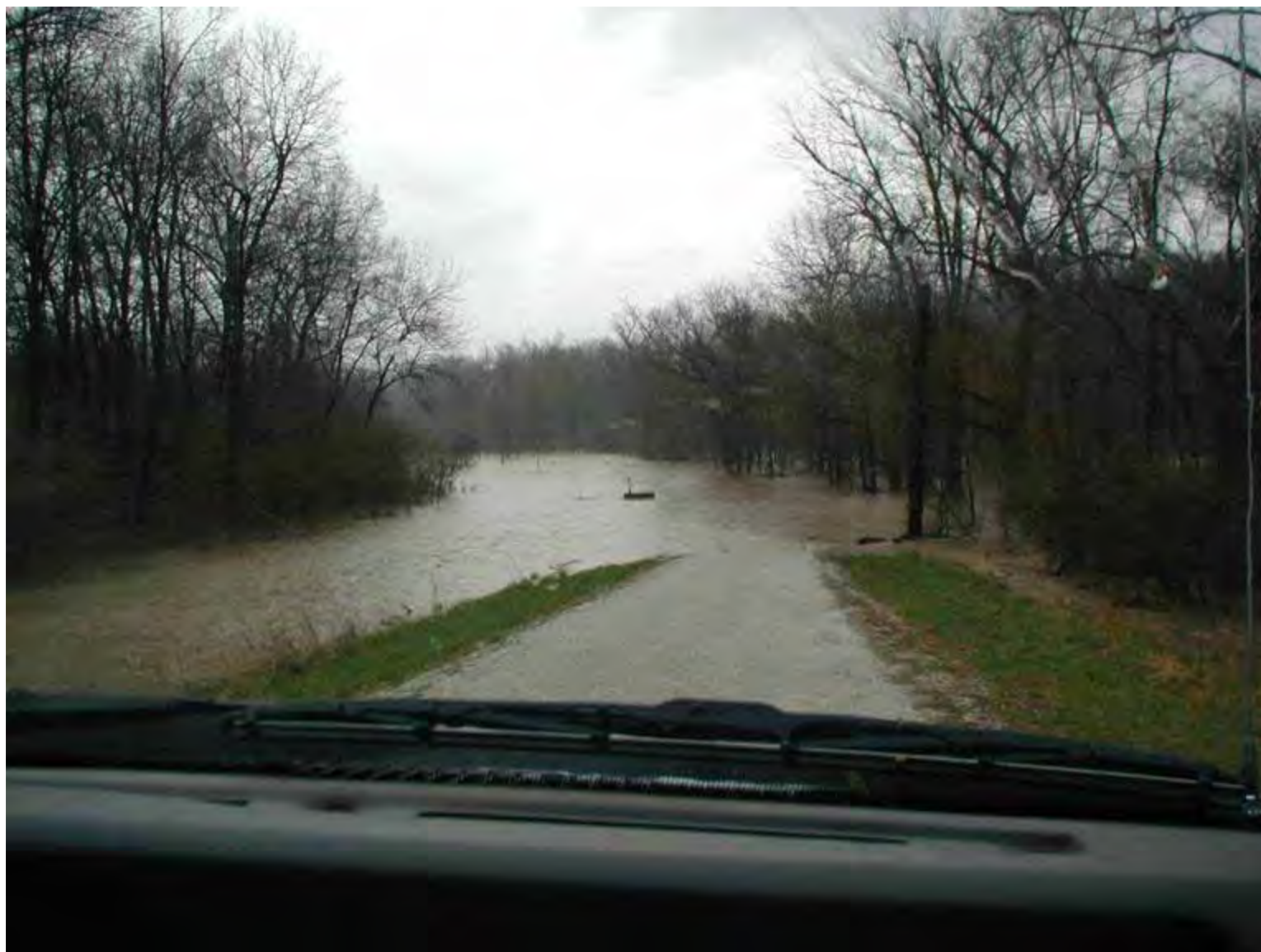
Bear Creek Trail during flood.
