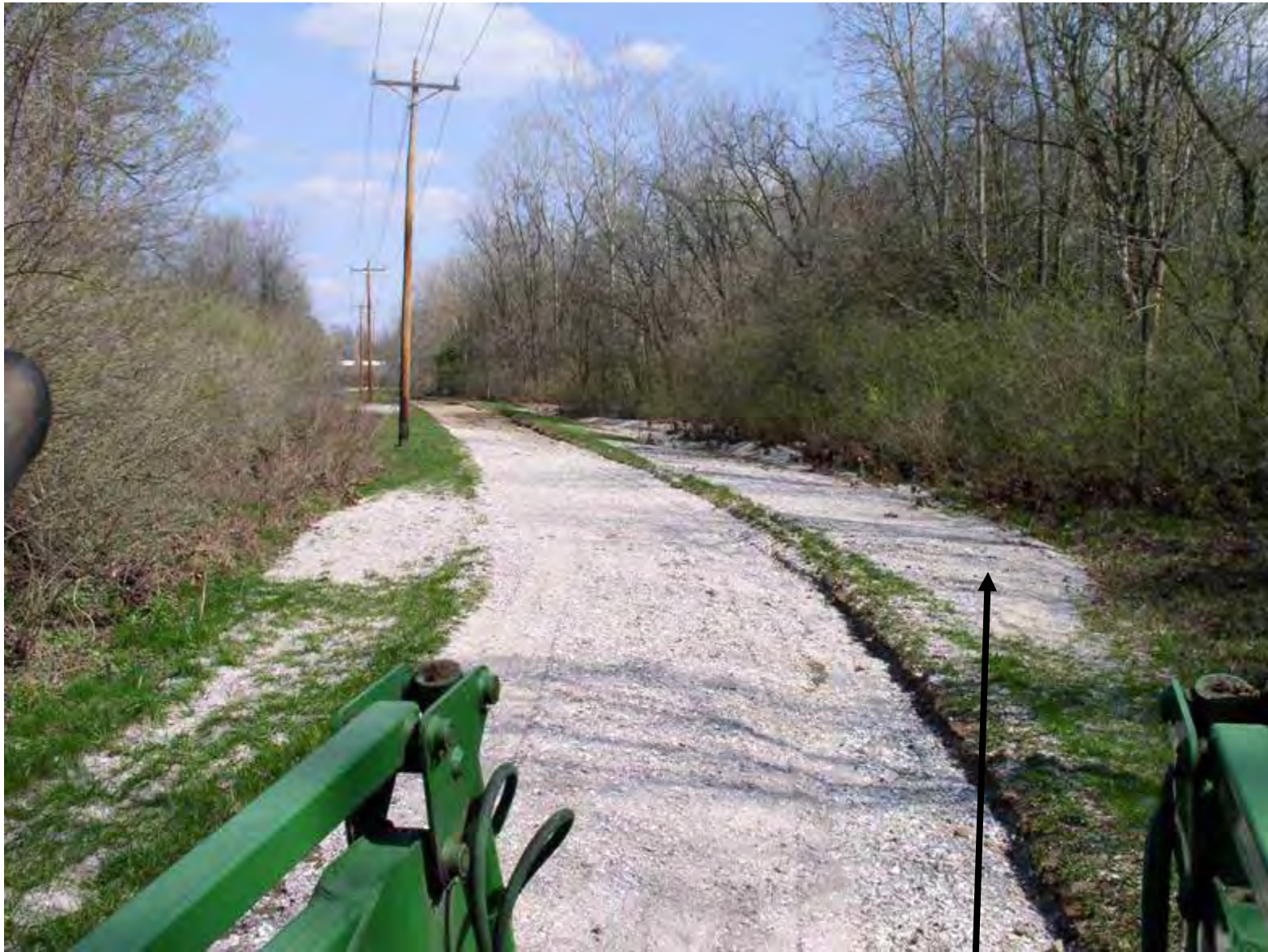
Gravel build-up in natural areas after flooding.
