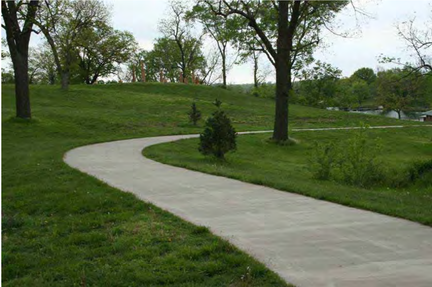
Stephens Lake Park 10' concrete trail
