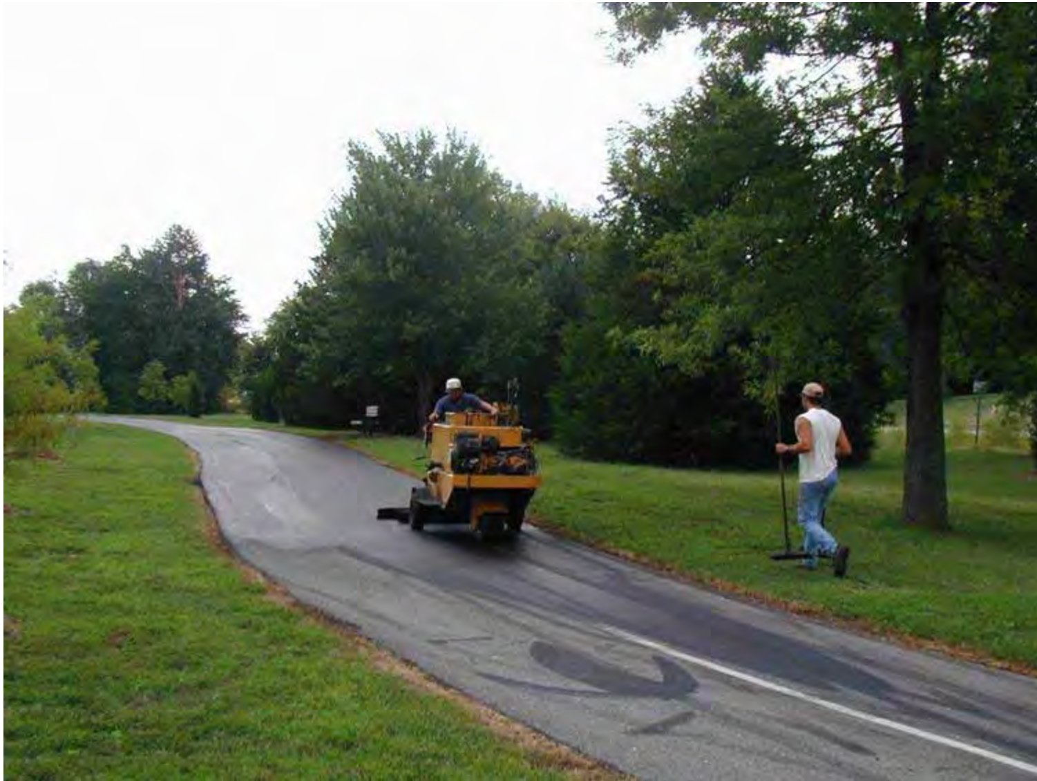
Cosmo Trail required crack filling and sealing after only 2 years.
