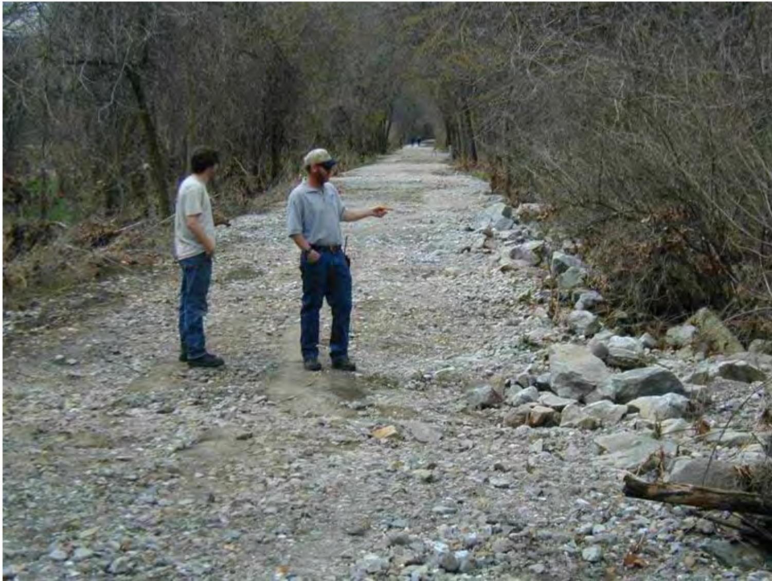
Replacing rock after flooding along the MKT Trail.
