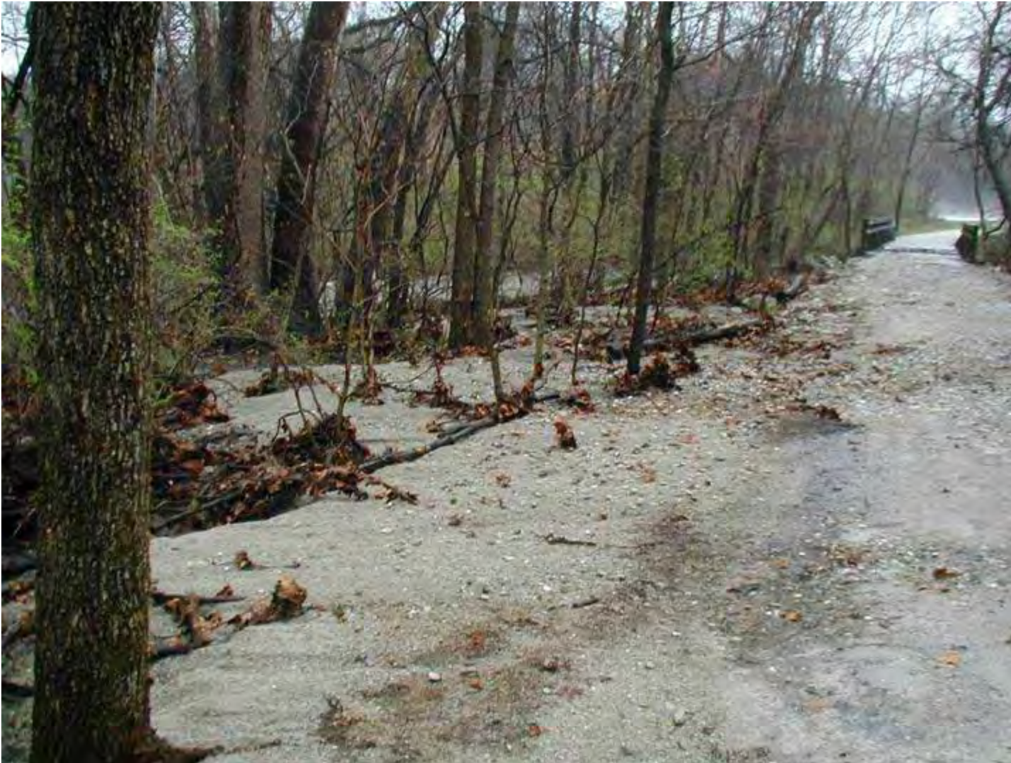
Gravel build-up in natural areas after flooding.
