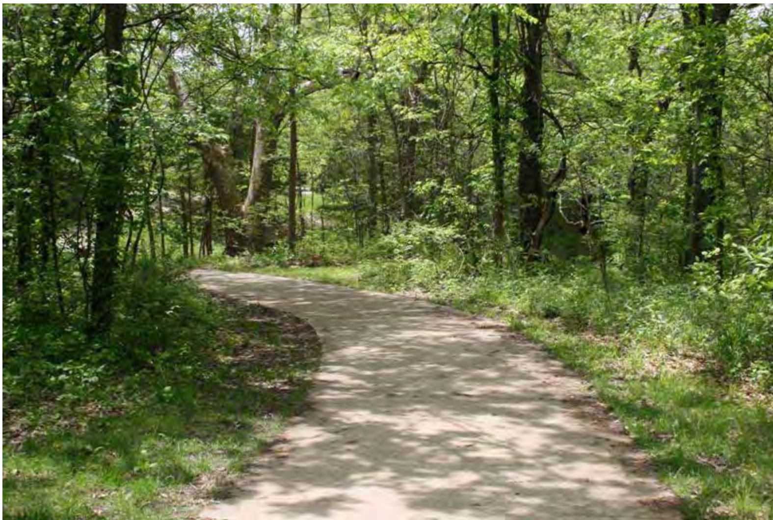
15 year old concrete in perfect shape at Oakland Park 8' trail.
