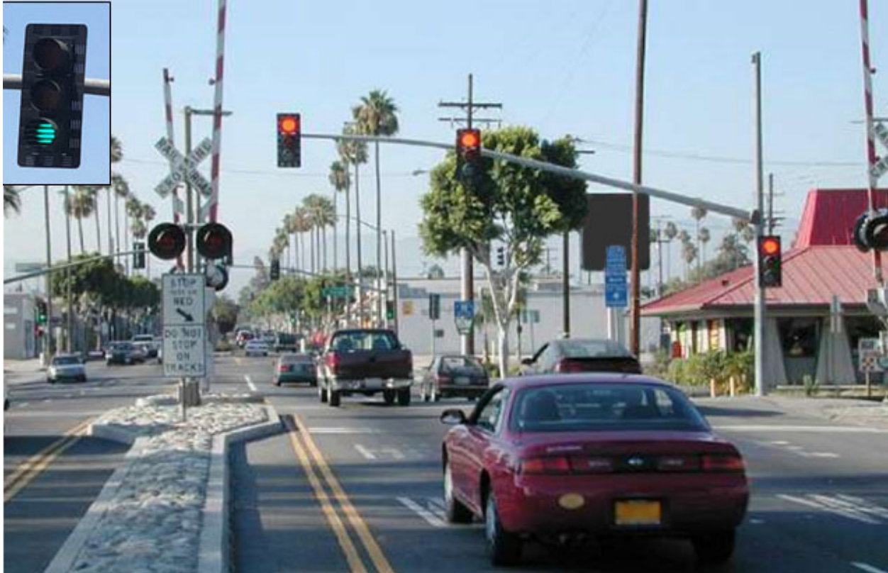
Figure 41. Illustrative Example Showing Downstream Mounted Pre-Signal (SCAX Sierra Avenue Crossing at Orange Way, Fontana, CA, USDOT 026145L)
