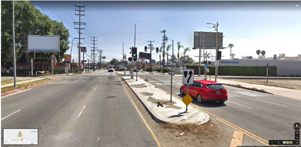
Figure 43. Illustrative Example of Queue Cutter (SCAX Balboa Boulevard Crossing at Roscoe Boulevard in Los Angeles, CA, USDOT 745989G)
