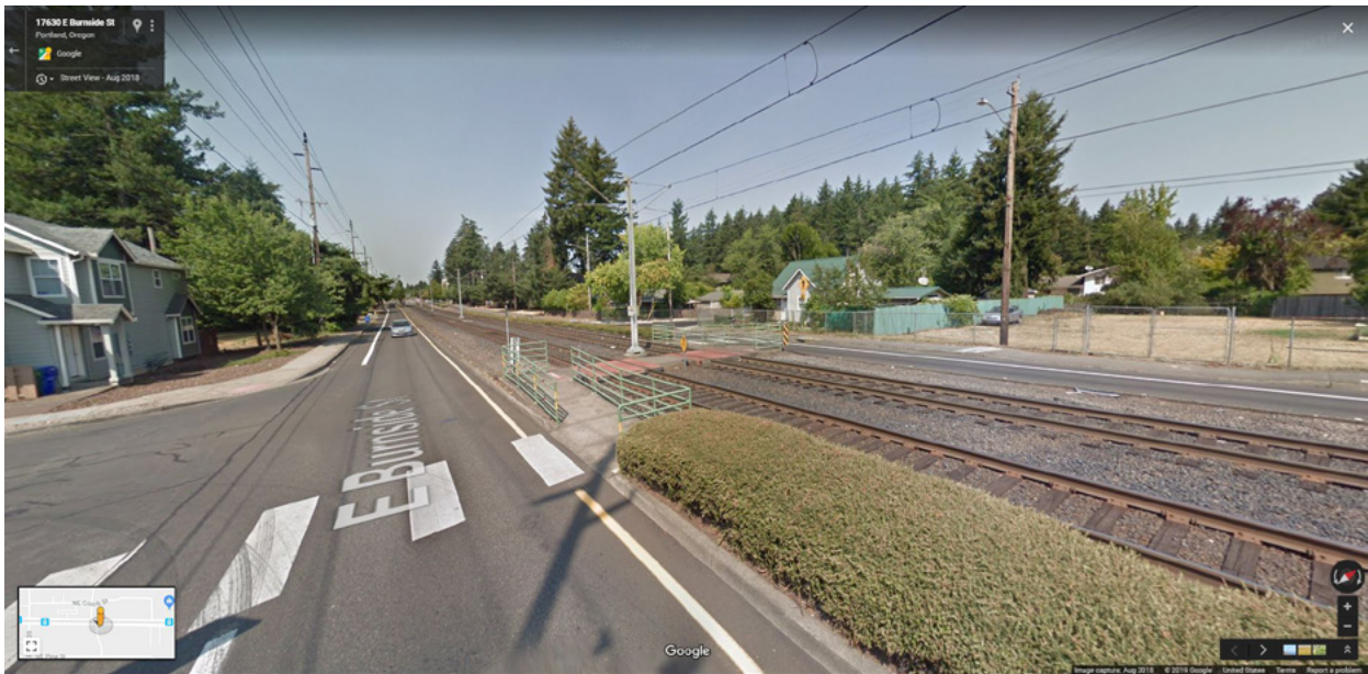
Figure 54. Illustrative Example of a Z-Crossing (Portland TriMet, Burnside Avenue, Portland, OR)
