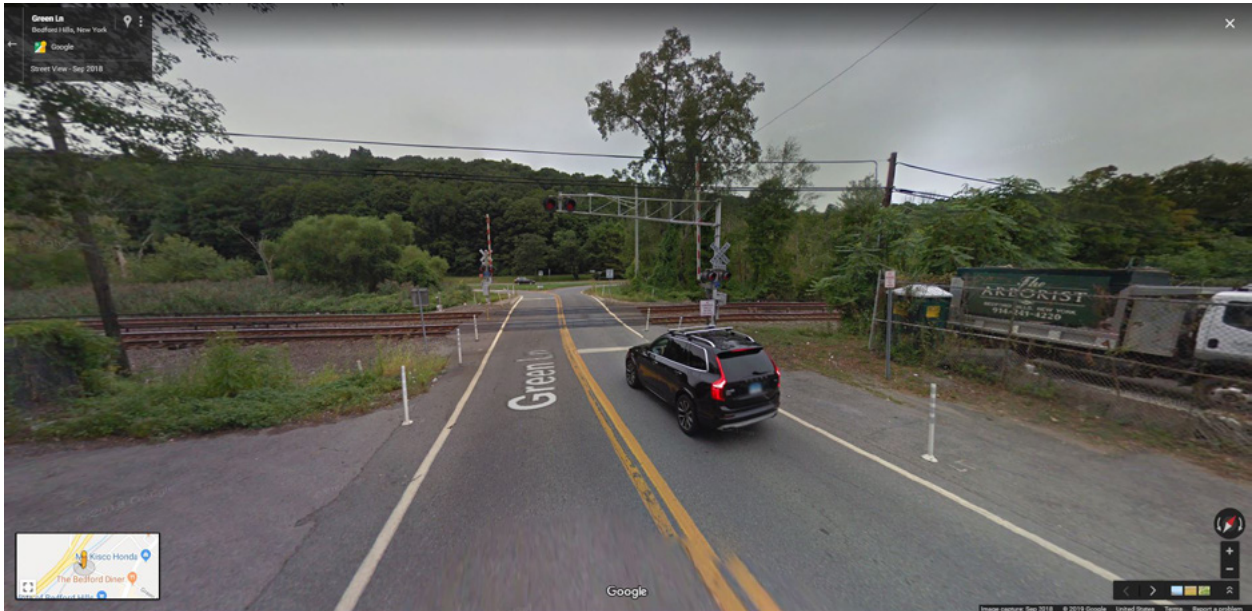
Figure 18. Illustration of Use of Tubular Markers (Metro North Harlem Subdivision, Green Lane Crossing, Bedford Hills, NY ID 529898H)
