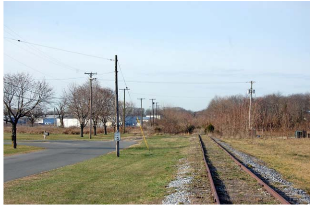
Inactive tracks looking west from Vine Road
