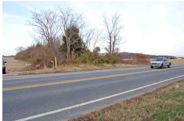
The abandoned Bridgeton Secondary crosses Big Oak Road in Upper Deerfield Township
