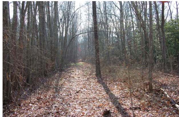
Abandoned PRSL Maurice River branch parallel to Newell Road south of Leesburg
