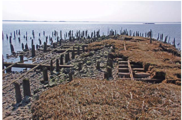
Abandoned CNJ railroad begins at Caviar Point within PSEG's Bayside Tract
