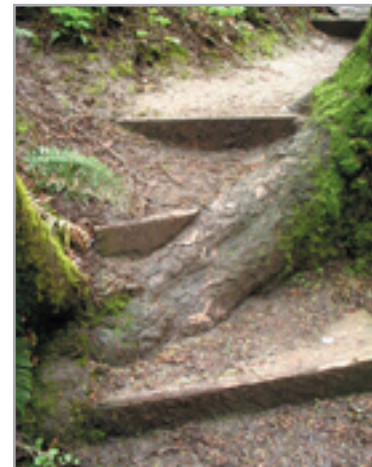
Marshall Park Trail - steps built around tree root
