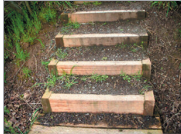
Dickinson Park - cribbed steps
