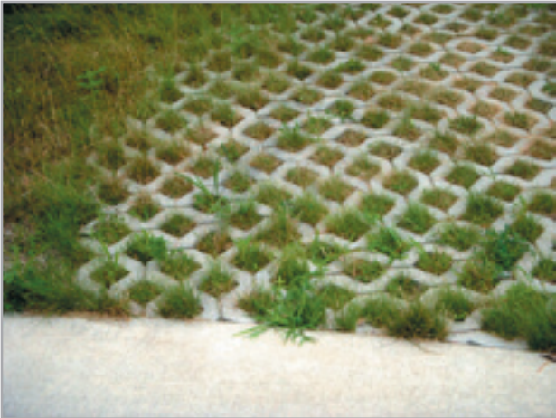
Concrete turf block used to provide maintenance access in Vancouver, B.C.
