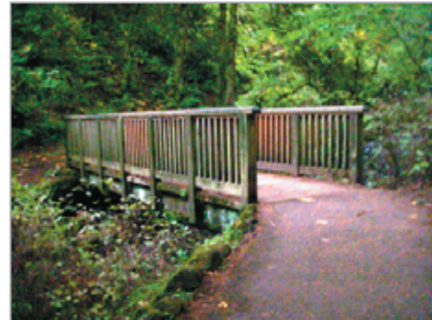
Balch Creek bridge on Lower Macleay Trail in Forest Park (part of an accessible trail) has balusters to prevent falls into creek
