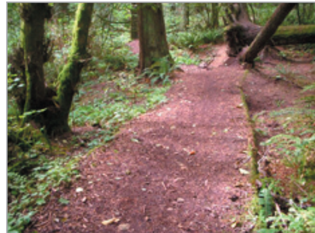
Wild Hawthorn Trail in Powell Butte - cedar log causeway in level, poorly drained area near base of bluff
