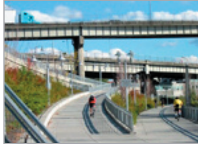
Vera Katz Eastbank Esplanade - accessible ramp near Riverwalk on Steel Bridge
