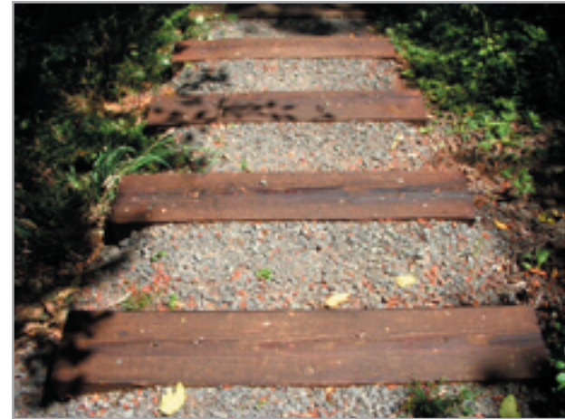
Raz-Baack crossing at Stephens Creek Nature Park - timber steps
