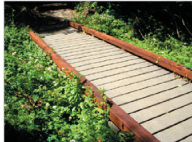
Raz-Baack crossing at Stephens Creek Nature Park - boardwalk with plastic lumber decking
