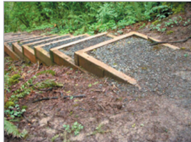
Woods Memorial Park - cribbed steps under construction
