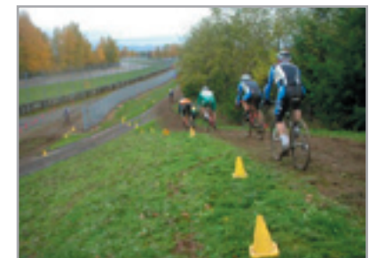
H - Levee and maintenance road
