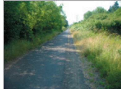
Springwater between Palmbled and Rugg Roads - one gravel shoulder widened for equestrian and runner use
