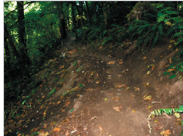
Connor Trail - rolling grade construction
