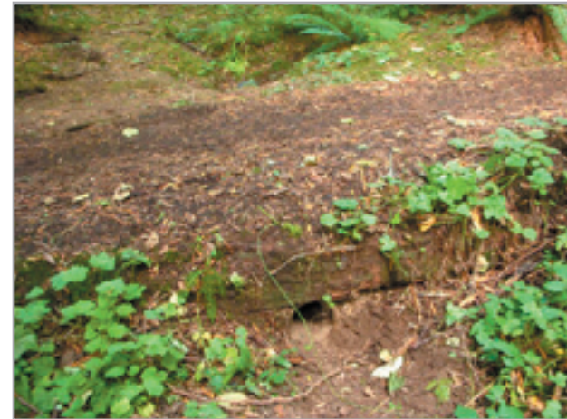
Wild Hawthorn Trail in Powell Butte - split cedar causeway and small drain pipe
