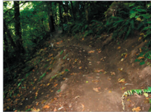
Connor Trail - rolling grade construction
