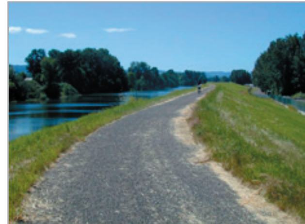
Columbia Slough Trail at PIR and Heron Lakes Golf Course - this segment is surfaced with chipseal, a product no longer used by PP&R due to its rough surface and lack of durability
