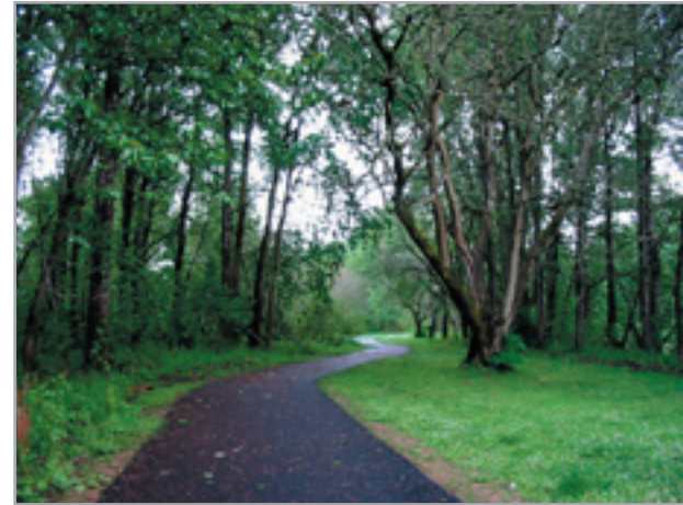
Kelley Point Park - newly installed porous asphalt trail
