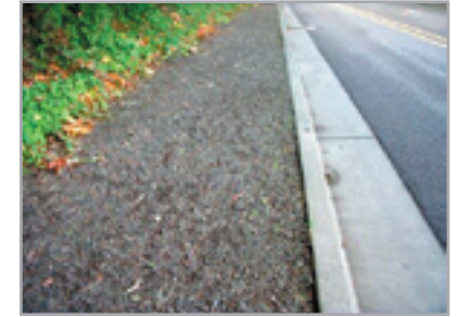
40-Mile Loop Trail at base of Forest Park’s Ridge Trail, next to Bridge Access Road for St Johns Bridge
