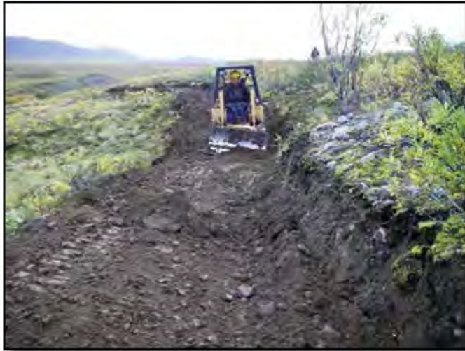
The Glacier Lake Trail was designed as a 7- to 8-foot wide tread with a full bench. The Sweco 480 is digging the grade down to native material to meet the full bench specification.
