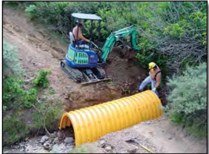
Figure 14–2—A miniexcavator is a versatile piece of equipment for trail construction and maintenance and plays a valuable role in supporting trail dozer operations.
