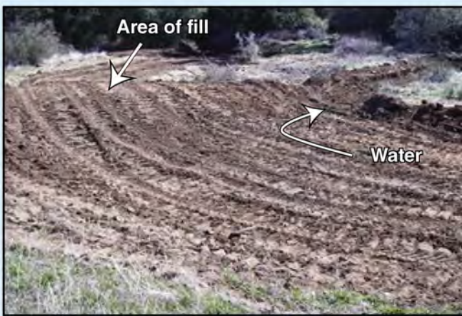
Figure 2–8—Rolling grade dips are constructed to direct water off existing trails.
