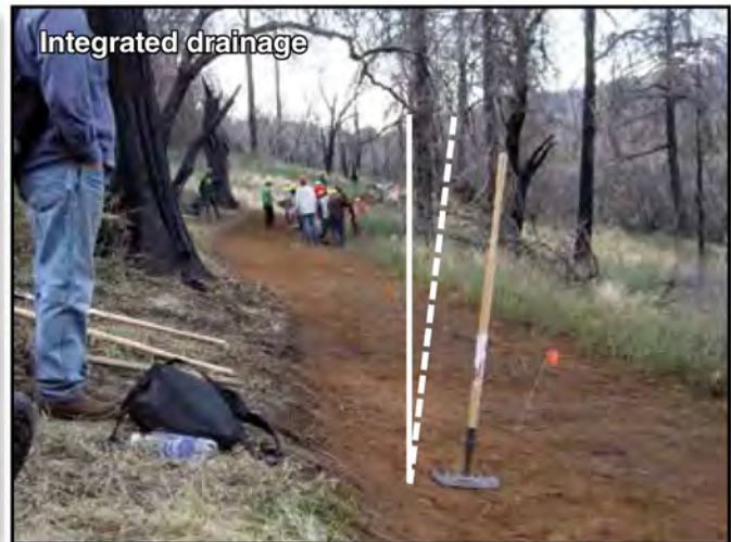
Figure 2-3—Note the angle of the trail tool handle. It shows that the trail tread has outslope, one type of integrated drainage (the third sustainable trail design guideline). Outslope encourages water to flow across the trail. Unfortunately, functional outslope is usually lost on off-highway vehicle trails when wheel ruts form. Grade reversals and rolling dips overcome this problem.
