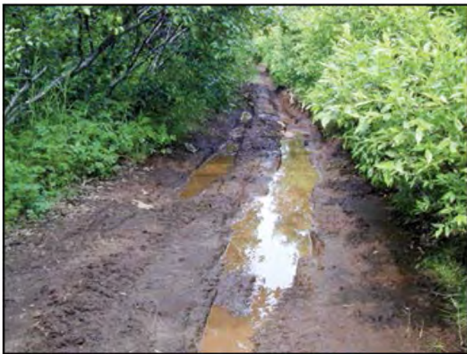
Figure 2–14—This trail on Alaska State land near Homer, AK, does not have permafrost, but the trail became muddy and rutted after traffic entrenched the trail relative to the surrounding terrain.
