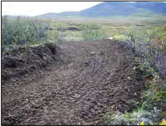
Superelevated (banked) turns also are integrated into the alignment. This design element reflects the heavy expected use of the trail by all-terrain vehicles (ATVs). The outside edge elevation works with the forces exerted on the tread by the ATVs as they traverse the turn.
