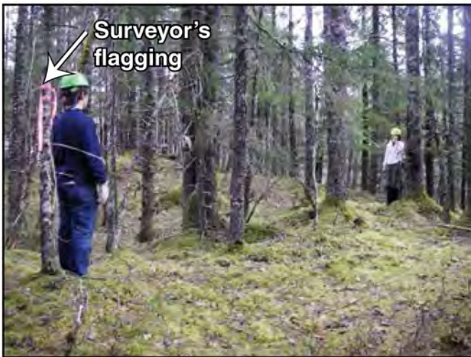
Figure 12–12—Surveyor's flagging is hung at the eye level of the person using the clinometer during trail layout.
