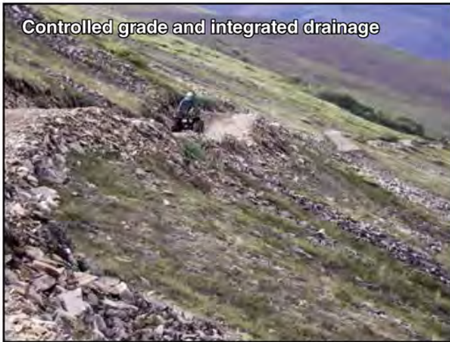
Figure 2-2—This off-highway vehicle trail in the Bureau of Land Management White Mountains National Recreation Area illustrates controlled grade and integrated drainage, the second and third sustainable trail design guidelines. Note how the trail slowly descends the sidehill. In this case, the grade never exceeds 10 percent and grade reversals (short, abrupt changes in grade) serve as integrated water control features. The all-terrain vehicle rider visible in the photo is traversing the bottom of one of the grade reversals.
