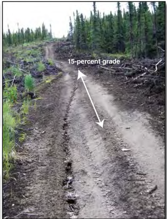
A portion of the ridgetop fireline used to access the Compeau trail. Note the fall-line alignment and lack of integrated water control—a few of the features that limit the sustainability of this adapted trail segment.
