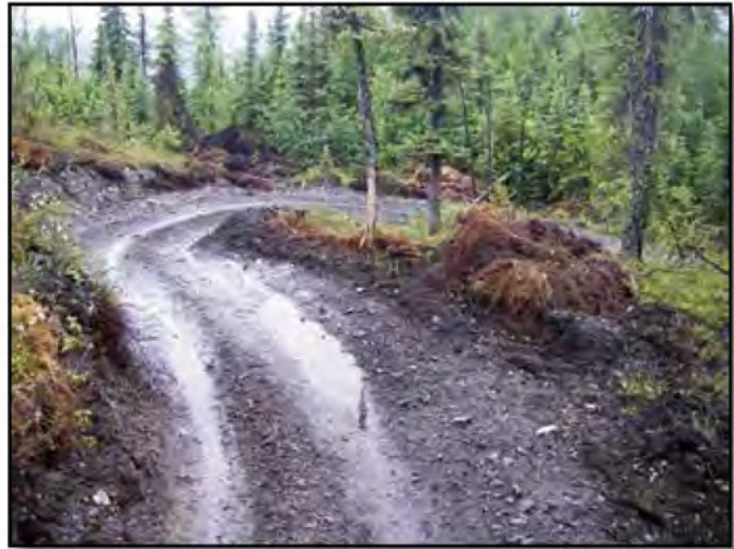
Figure 13–1—Off-highway vehicle (OHV) traffic on this cut-through climbing turn quickly forms wheel ruts and banked turns that can disrupt tread surface drainage. Regrading these to their original specifications is one of the primary purposes of OHV tread maintenance.
