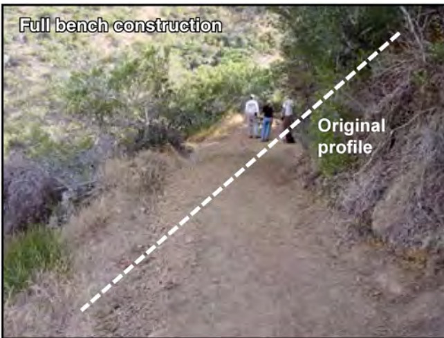
Figure 2-4—This profile of a Catalina Island, CA, foot trail illustrates full bench construction, the fourth sustainable trail design guideline. The dashed line indicates the original profile of the sideslope. Note how the entire slope has been excavated to ensure that the trail tread is supported by the most durable tread surface possible.
