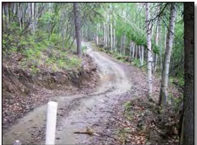
One of the many grade reversals integrated into the trail alignment to make sure that water flows on average for no more than 100 feet along the tread surface.
