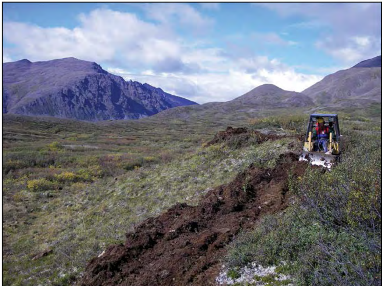
A Sweco 480 trail dozer roughs out the trail bench on the Glacier Lake Trail above Rock Creek. The Sweco 480 is specially designed for trail work. It has a track width of 4 feet and a six-way blade that is 5 feet wide. Jon Underwood of Happy Trails, Inc., Fairbanks, AK, was the owner/operator for the project excavation.
