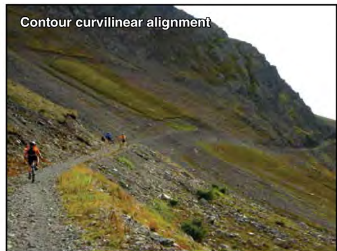
Figure 2–1—This trail in the Chugach National Forest illustrates contour curvilinear alignment, the first sustainable trail design guideline. Note how the trail crosses the slope along the topographic contour rather than running more directly up or down the slope. The sideslope location of the trail and its alignment encourage the natural force of gravity to carry water across the trail rather than directing it down the trail.
