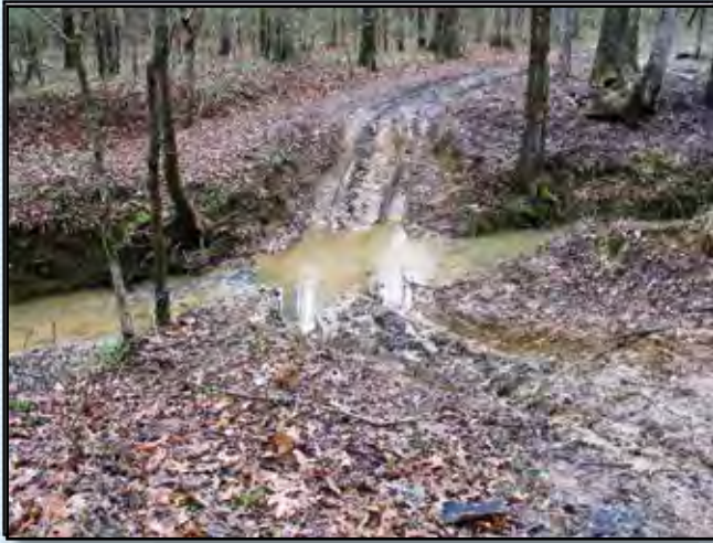
Figure 7-4—Degraded water crossings can harm water quality.
