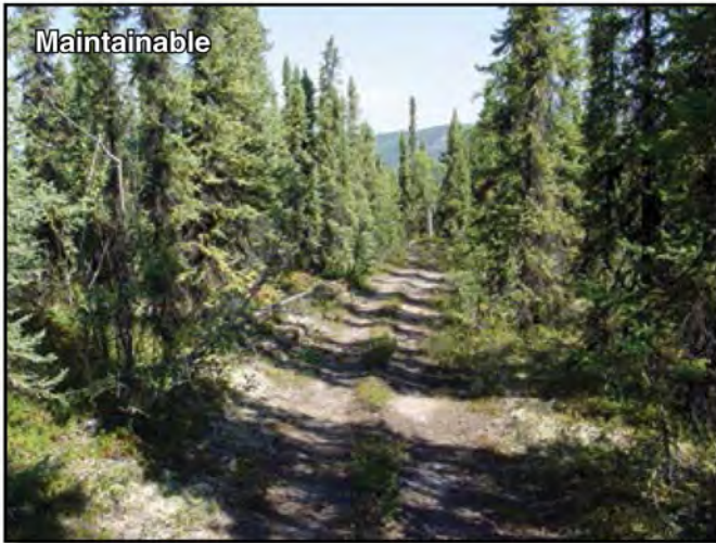
Figure 3-3—An example of a maintainable trail section in the Fortymile River area, AK. This section has a contour alignment and an average trail grade less than 10 percent, but it lacks adequate water control. Rolling grade dips could be integrated into the alignment for increased sustainability.
