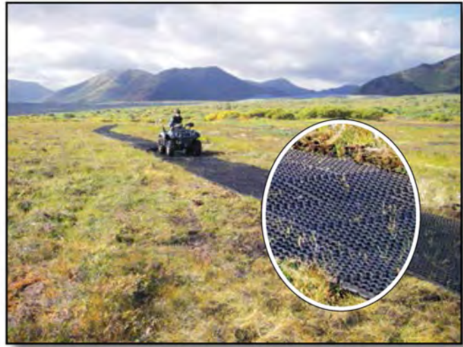
Figure 11–7—A trail-hardened surface of porous pavement panels provides passage over permafrost-associated wetlands on the Karluk River Portage Trail within Alaska’s Kodiak Island National Wildlife Refuge.
