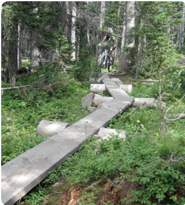
**Elevated Tread.** A puncheon / bog bridge used to cross wet area with minimal impact and add interest to trail near Brainard Lake, CO.
