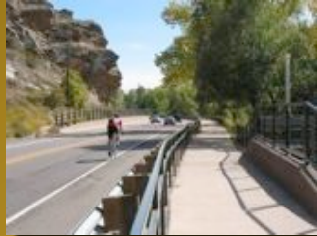
Custom Pedestrian Railing protecting trail users from back of guardrail
