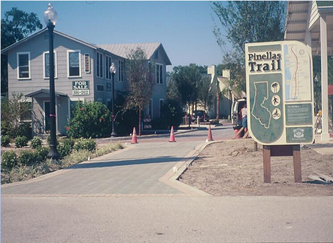
Trail under construction
