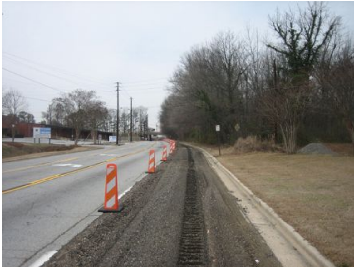
Road Milling during Trail Construction.
