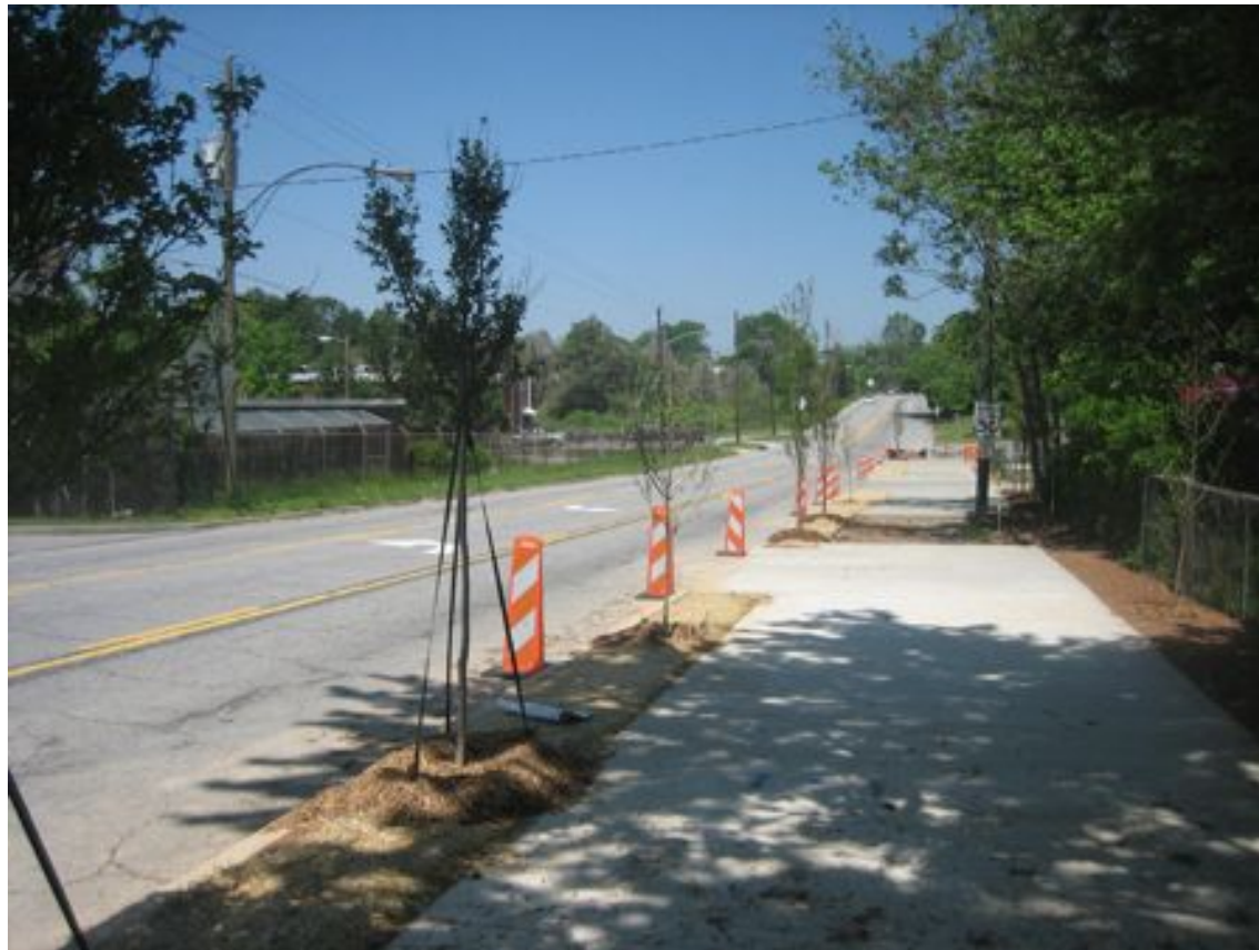
Challenges with Utility Relocation within Trail Corridor.
