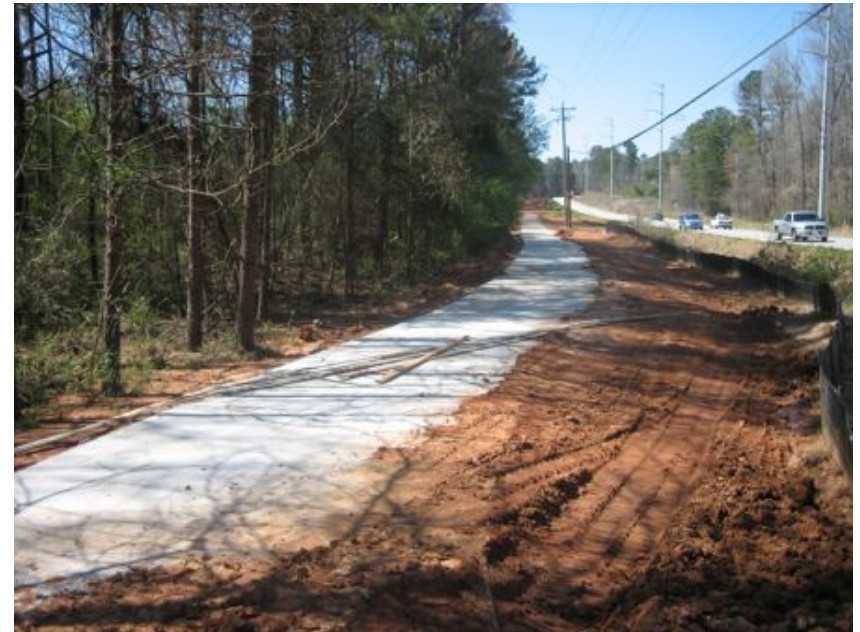
Trail Construction within existing Road Right-of Way.
