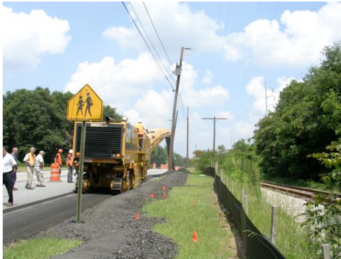
Construction of Multi Use Trail between Railroad and Road.
