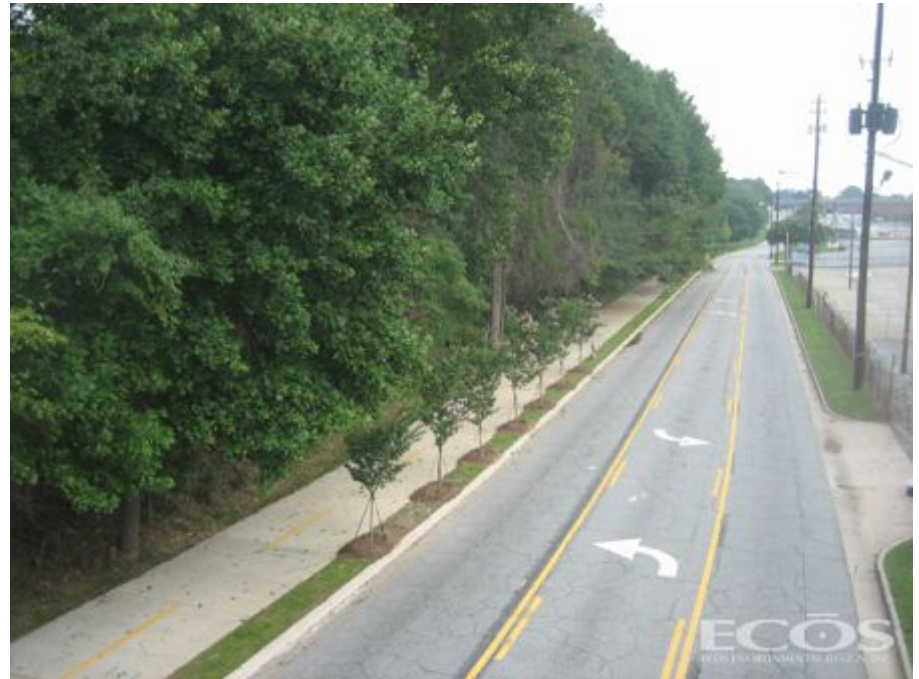
After – White Street (two lanes, turn lane and trail).
