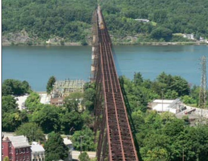
The bridge structure is visible as railroad tracks are removed
