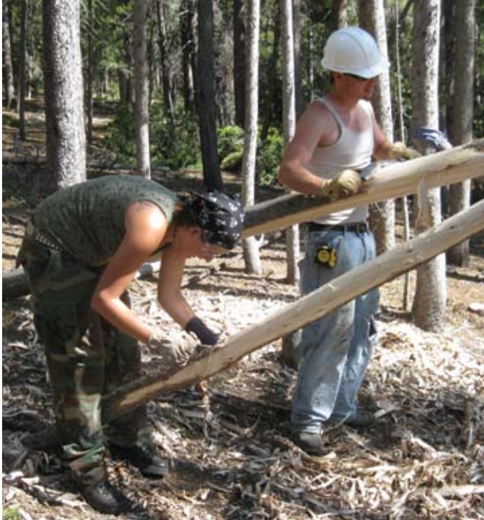
Peeling logs is the first step in backcountry construction
