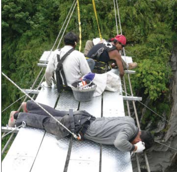
Workers extending the bridge section by section, while suspended over the gorge
