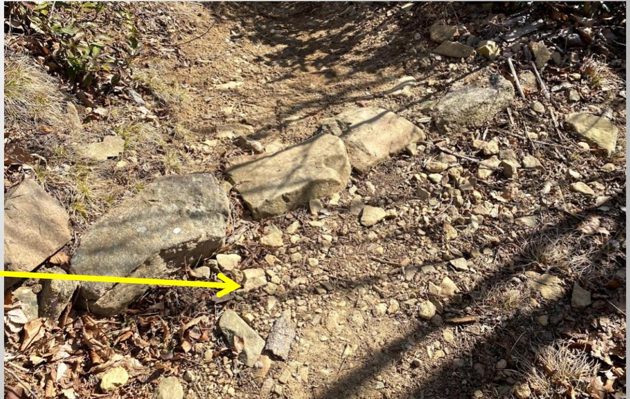
If a water bar does not have a **drain** to carry the water away from the water bar, the water slows down or stops and drops its sediment load. The area uphill of the bar silts up, and then the water just goes over it.
