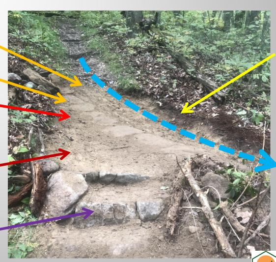
Sweeping curved drain and water bar routes water off trail without water slowing down and dropping sediment in drain.
