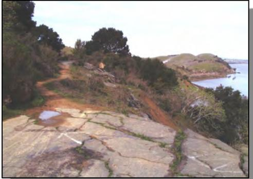
Segment 5080 on Carquinez Scenic Drive in Contra Costa County is a good example of a physical and financial constraint. The slope failure shown here is a physical constraint, while the funds required to fix it represent a financial constraint.
