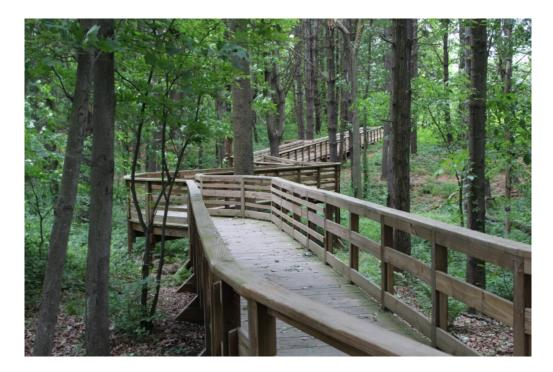
10. The two bridges are constructed in a similar manner. However, five 2" x 12s" were used as the stringers and the cross supports (2" x 12") and pads (3" x 3' x 4') are much more substantial.
