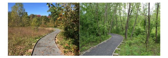
7. Small wooden openings along the sides of the trail are called "critter crossings" (escape passages); allowing small toads, snakes, and turtles to escape the path before they become dinner. They are generally located on the outside of the bends in the trail. The height is designed to meet ADA standards for the visually impaired while allowing critters to pass through. These escape hatches also provided the added benefit of draining water from the trail during large rain event.
