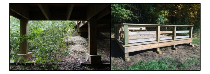
9. The entire trail is built on top of the ground. The wood structures use a combination of wooden pads rather than digging holes, to preserve the Native American artifacts that may be beneath the soil. Each elevated walkway is supported on 4" x 4" pressure treated posts that are resting on wooden pads. They were constructed in a series of 16' sections that include four (2"x8") pressure treated wood stringers supported every
