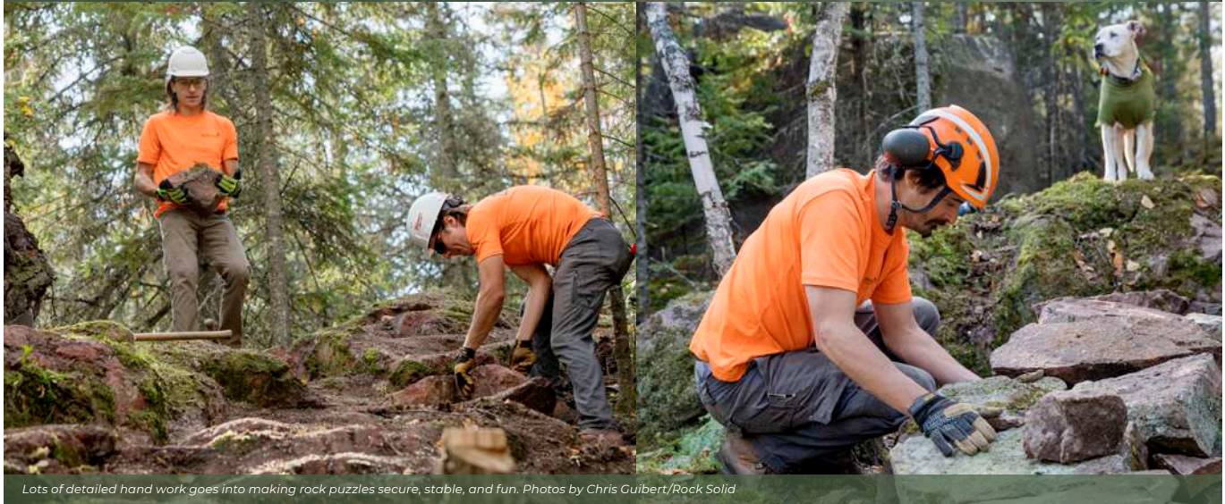
Rock drill prep for using feathers and wedges to split rock. Photos by Eli Glesmann/Rock Solid
