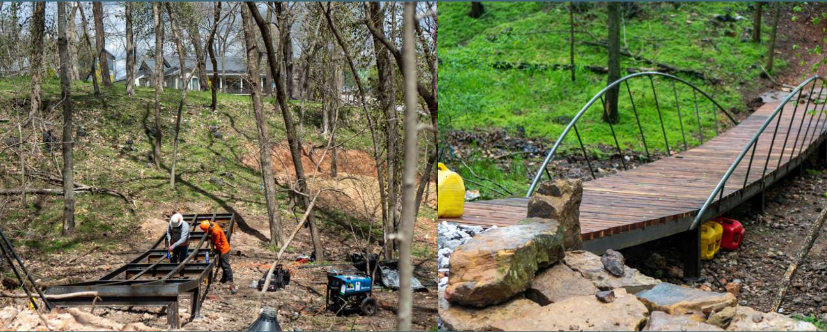
Steel-framed bridge with wooden decking at Headstart to Slaughter Pen in Bentonville, Arkansas. Photos by Eli Glesmann/Rock Solid
