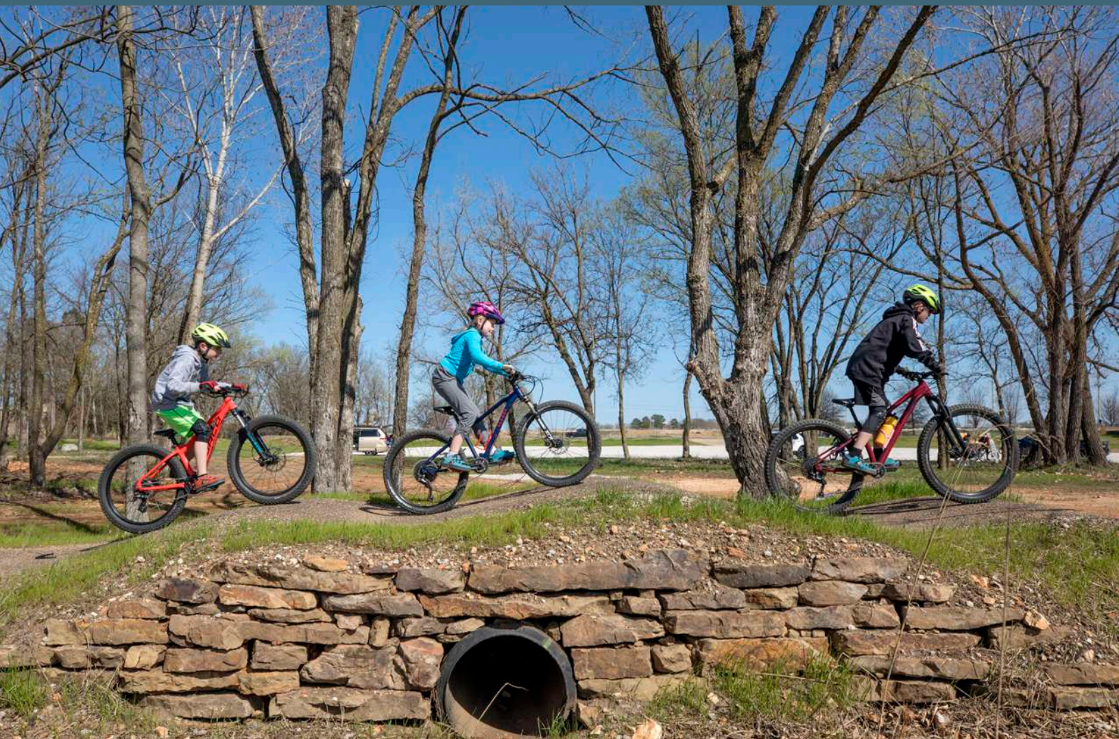
Roller section on Mama Bear chip-seal pump trail in Bentonville, Arkansas. Photos by Chris Guibert/Rock Solid
