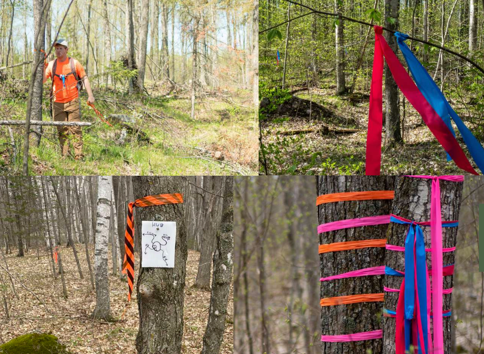
Flagging trail corridor, turns, and hubs in Marinette County, Wisconsin. Photos by Eli Glesmann/Rock Solid
