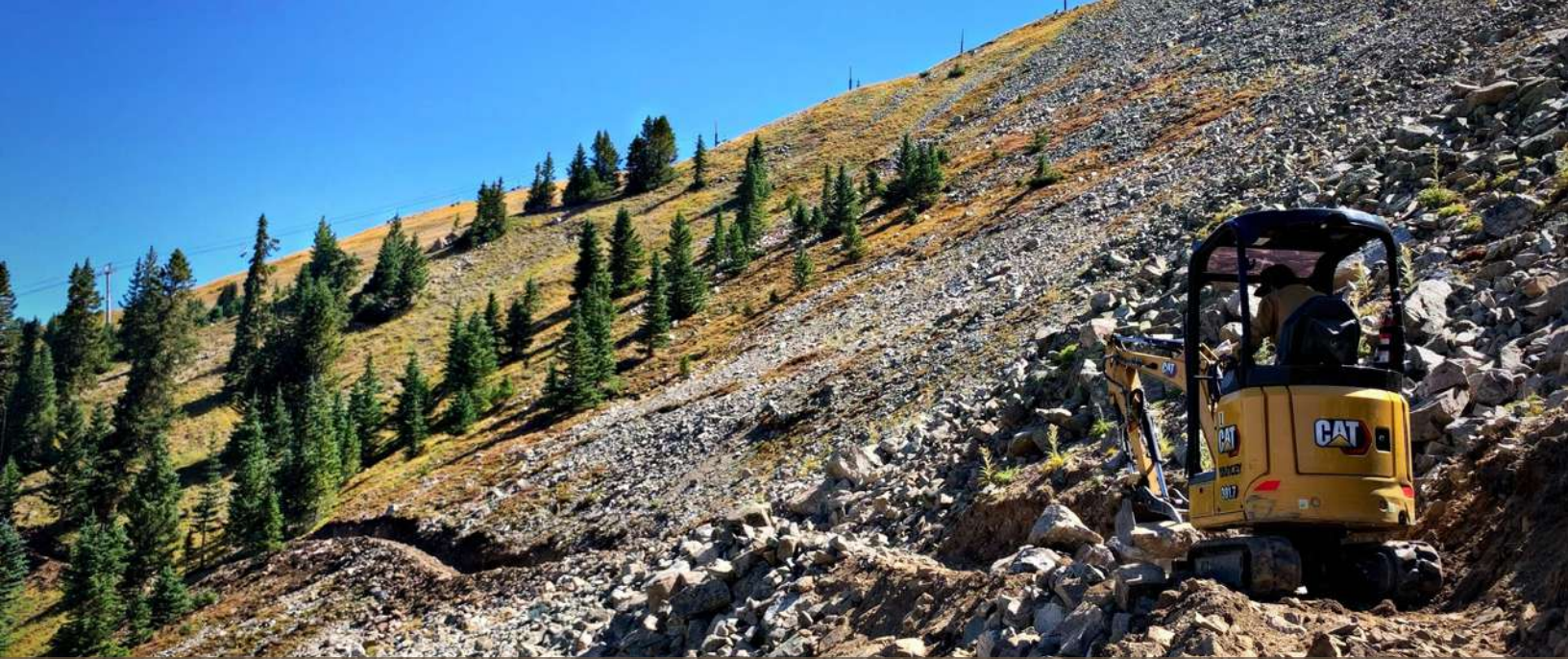
Excavator work at Arapahoe Basin, Colorado. Photo courtesy of IMBA
