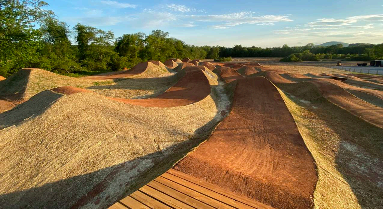
Progressive sets of dirt jump lines at Riveter in Fletcher, North Carolina. Photo courtesy of McGill Trail Fabrication
