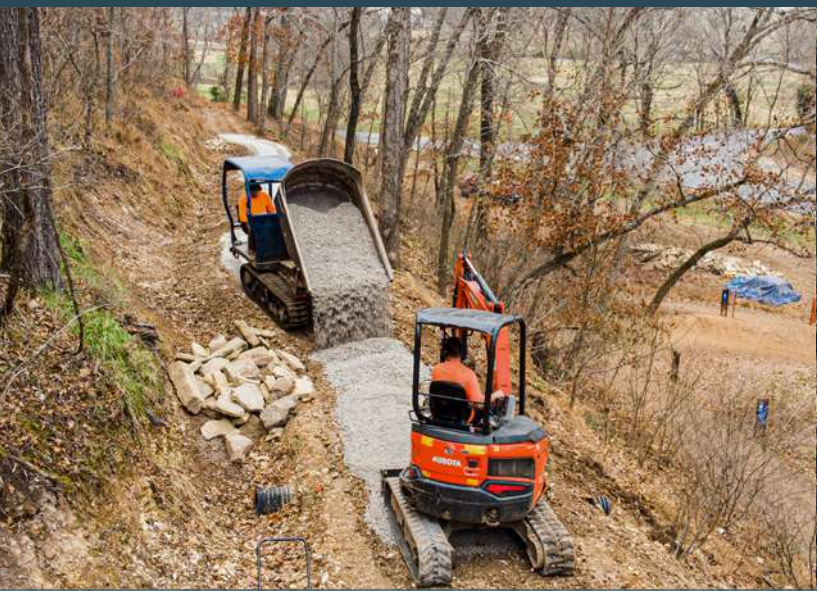
Chip-seal climb trail under construction at Coler Mountain Bike Preserve in Bentonville, Arkansas. Photo by Eli Glesmann/Rock Solid
