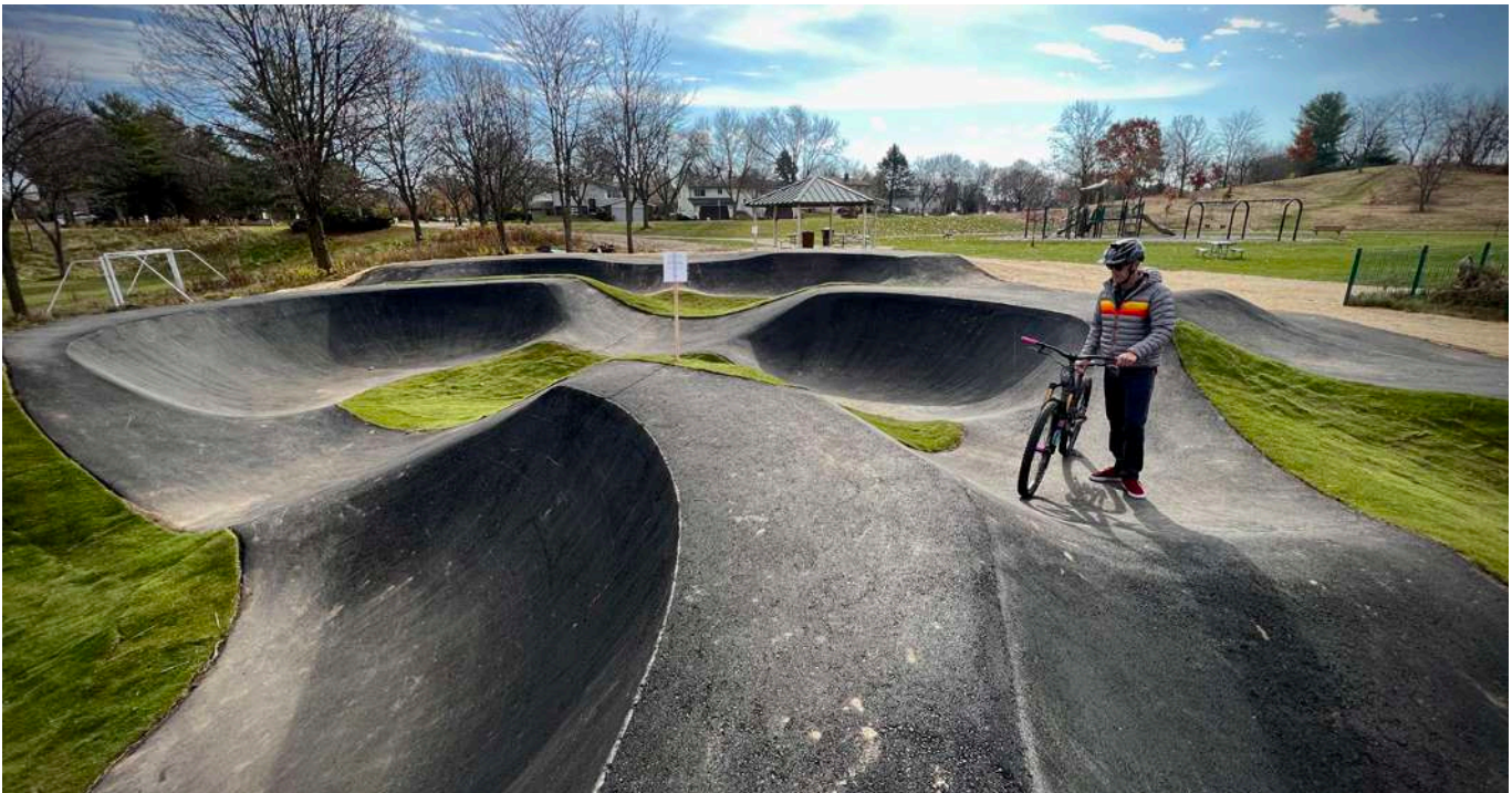
Asphalt-surfaced pump track at the Saris Foundation Bike Park at Aldo Leopold Park in Madison, Wisconsin. Photo by Repyak/IMBA
