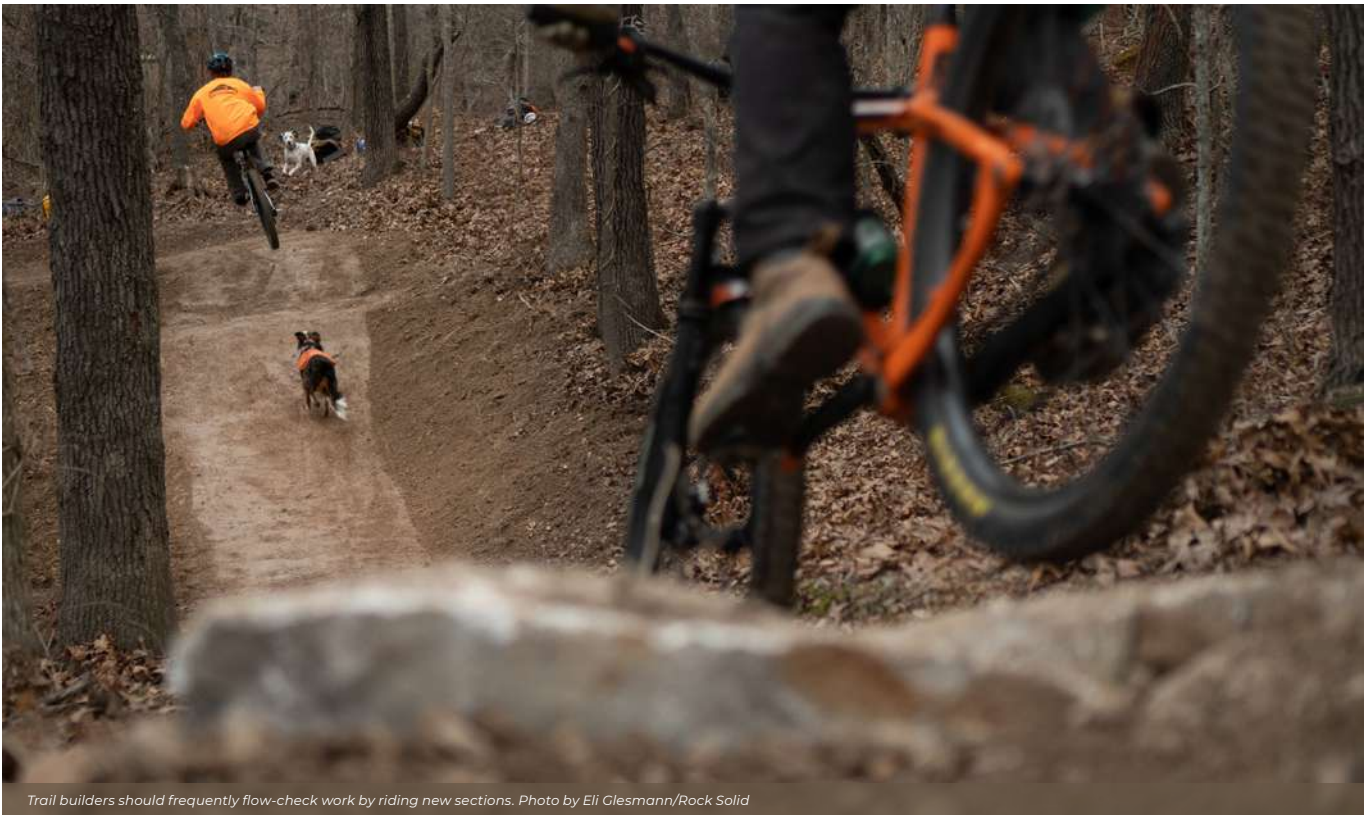
Trail builders should frequently flow-check work by riding new sections. Photo by Eli Glesmann/Rock Solid
