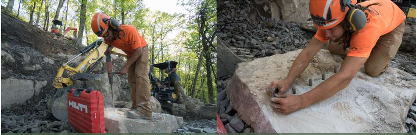
Rock drill prep for using feathers and wedges to split rock. Photos by Eli Glesmann/Rock Solid
