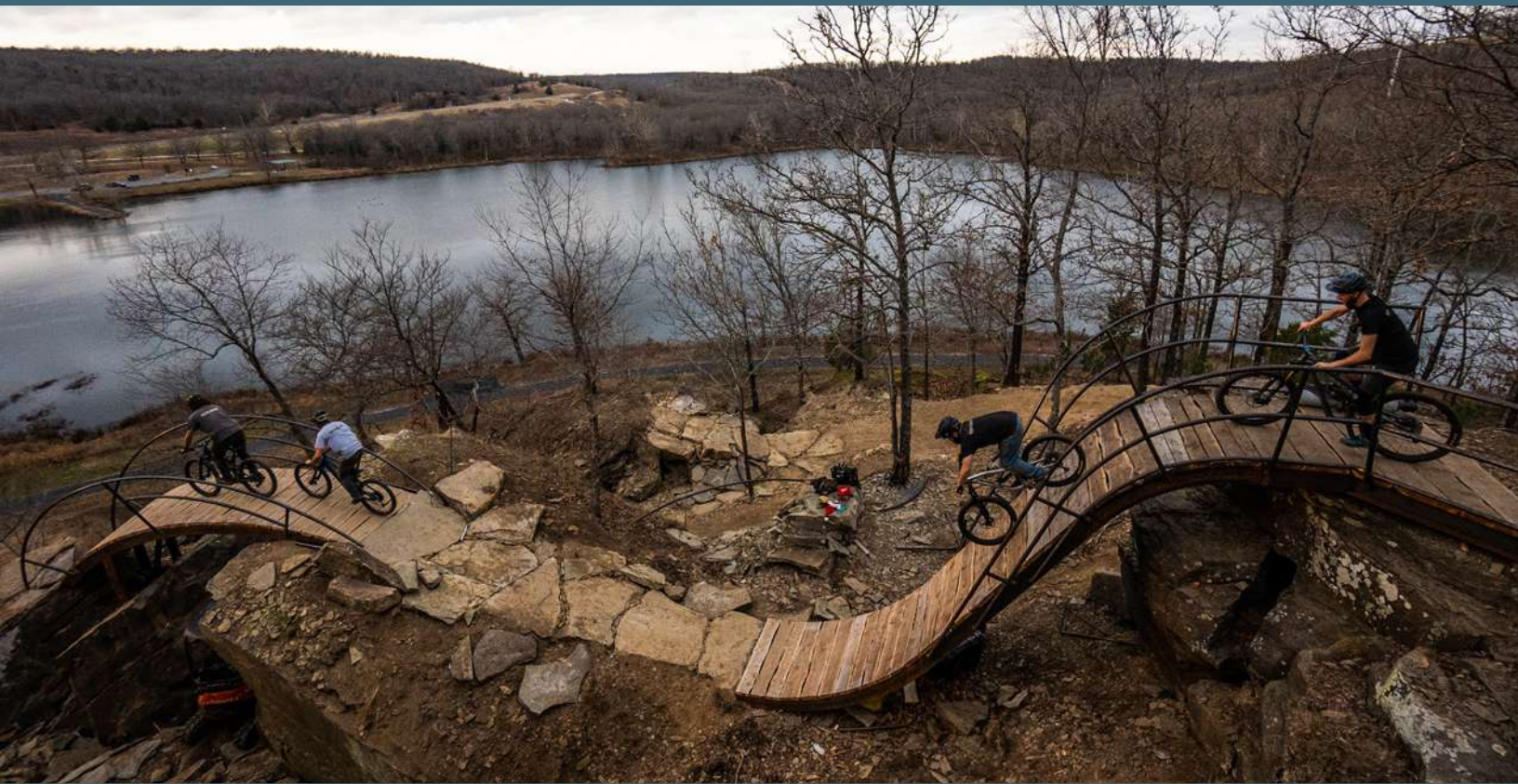
One-of-a-kind trail feature custom-designed and engineered to connect a cliff wall to a large rock "lily-pad" at Lake Vian in Vian, Oklahoma. Photo by Eli Glesmann/Rock Solid
