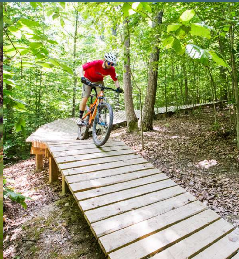
Wooden boardwalk with a canted turn for bike optimization. Photo courtesy of BLM/IMBA
