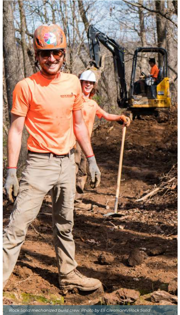
Rock Solid mechanized build crew. Photo by Eli Glesmann/Rock Solid
