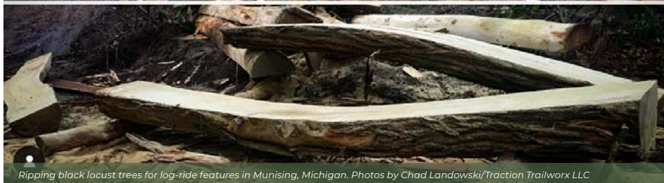
Ripping black locust trees for log-ride features in Munising, Michigan. Photos by Chad Landowski/Traction Trailworx LLC
