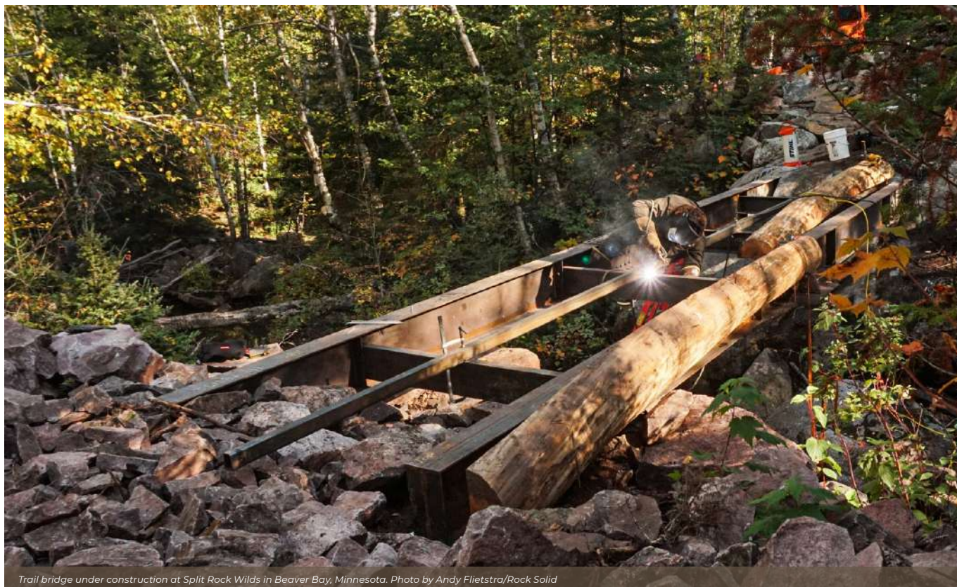
Trail bridge under construction at Split Rock Wilds in Beaver Bay, Minnesota. Photo by Andy Flietstra/Rock Solid
