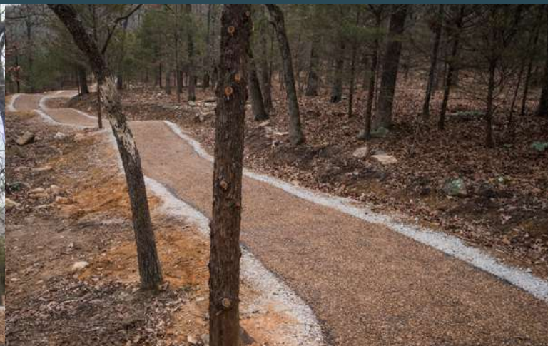
Freshly top-coated trail with liquid asphalt and small aggregate layers at Centennial Park in Fayetteville, Arkansas. Photo by Eli Glesmann/Rock Solid
