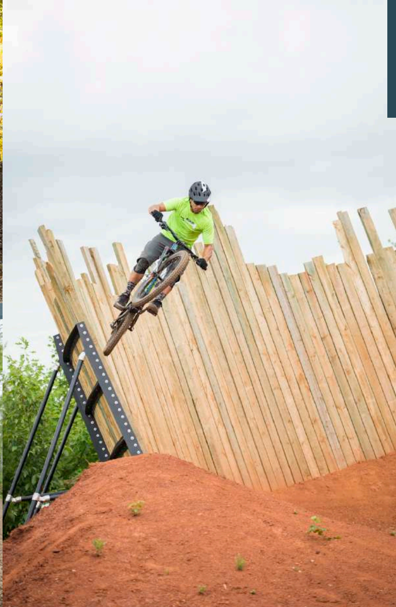
Slopestyle trail with constructed features on Devil's Racetrack in Knoxville, Tennessee. Photo courtesy of IMBA
