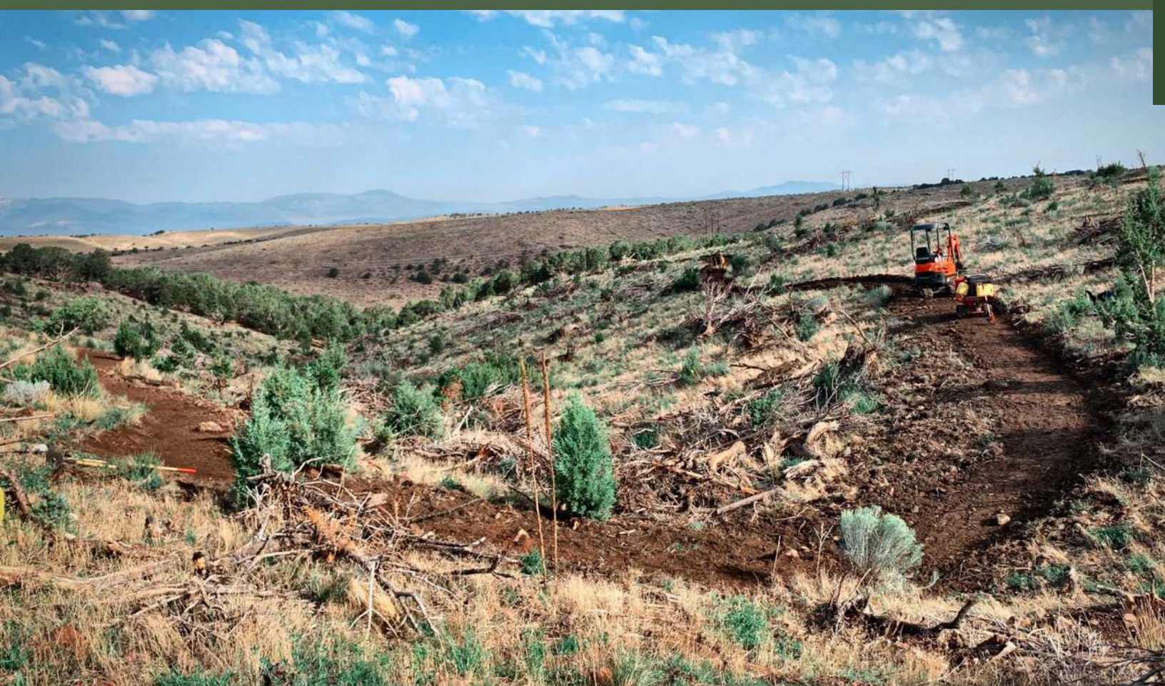
Tread construction in Cedar City, Utah. Photo courtesy of IMBA
