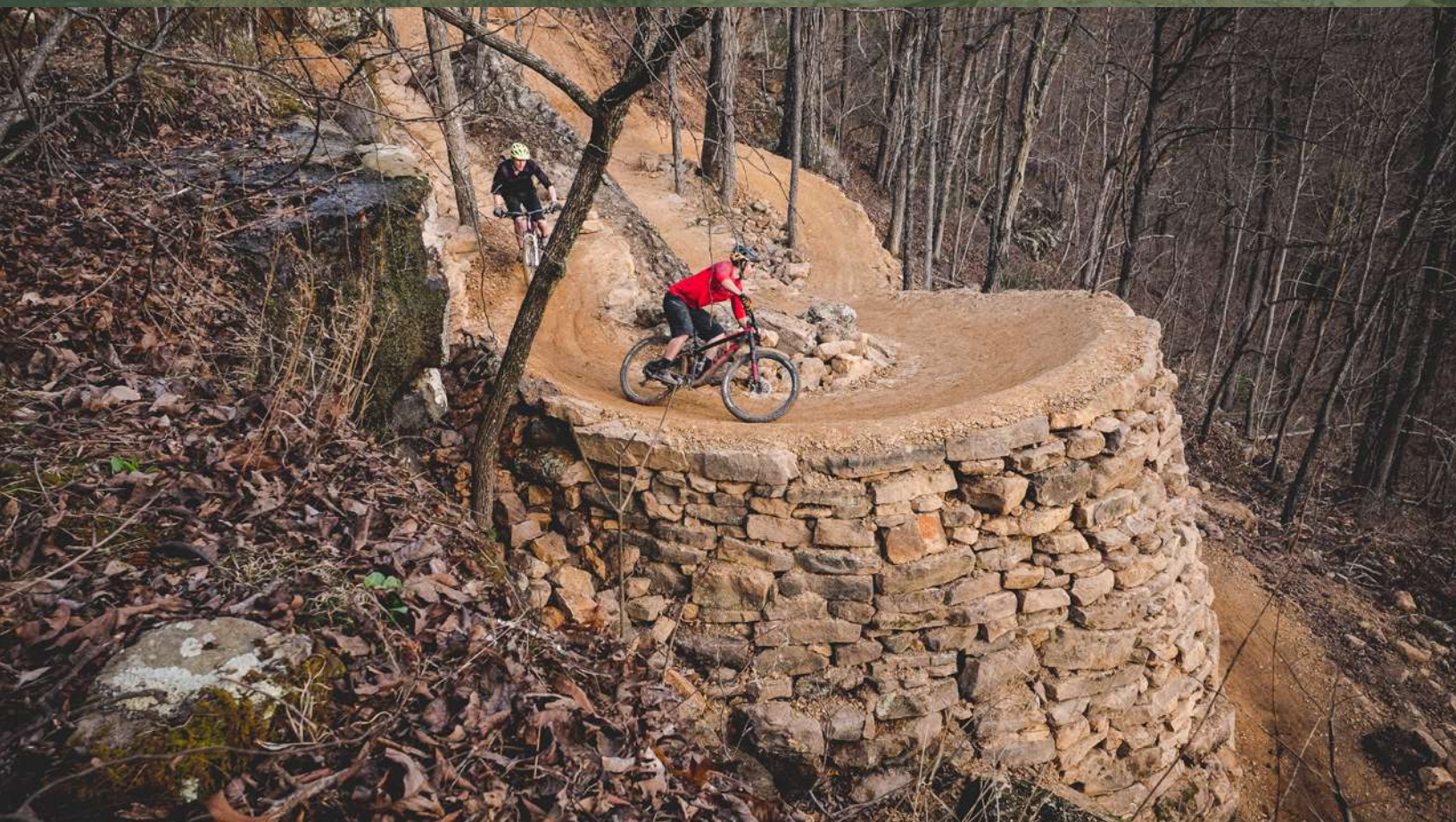
Construction of an extreme retaining wall was necessary to build the trail down a cliff wall. Photo by Hansi Johnson
