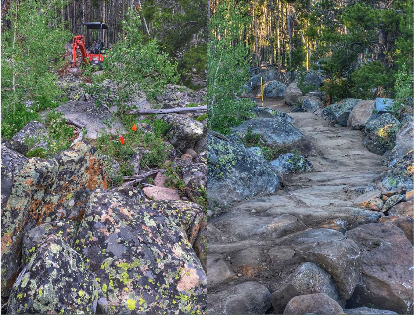
Before and after rock tread construction at Sinks Canyon in Lander, Wyoming. Photos by Adam Buck/Pathfinder Trail Building
