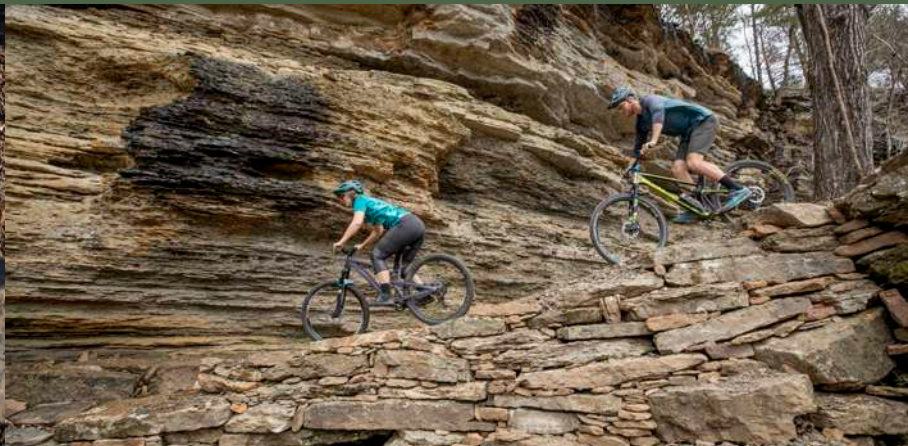
Intricate retaining wall at Devil's Den State Park in Winslow, Arkansas. Photo by Eli Glesmann/Rock Solid
