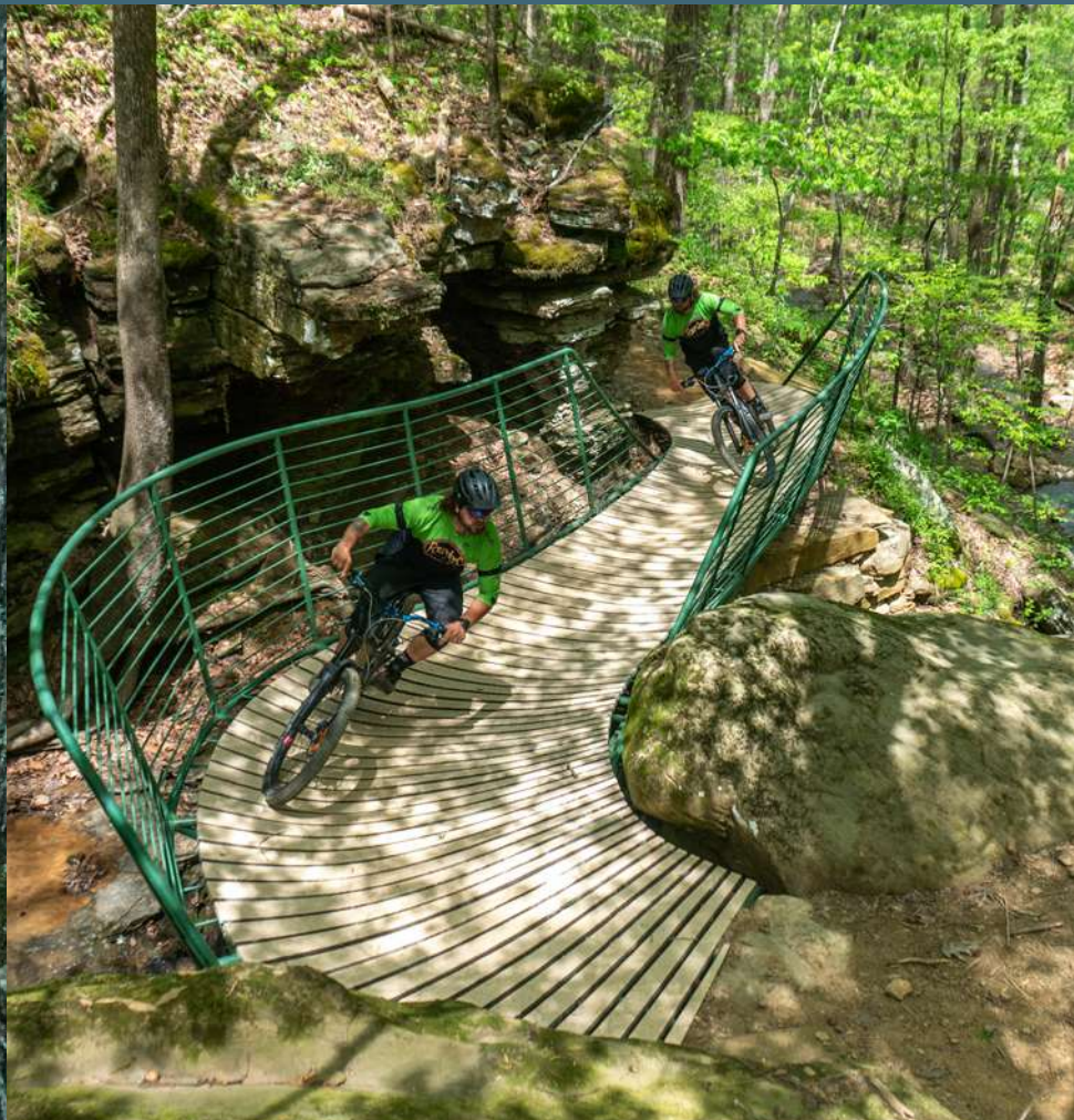
Complex, custom-engineered and site-built steel framed bridge at Mount Nebo State Park in Dardanelle, Arkansas. Photo by Andy and Michelle Flietstra/Rock Solid
