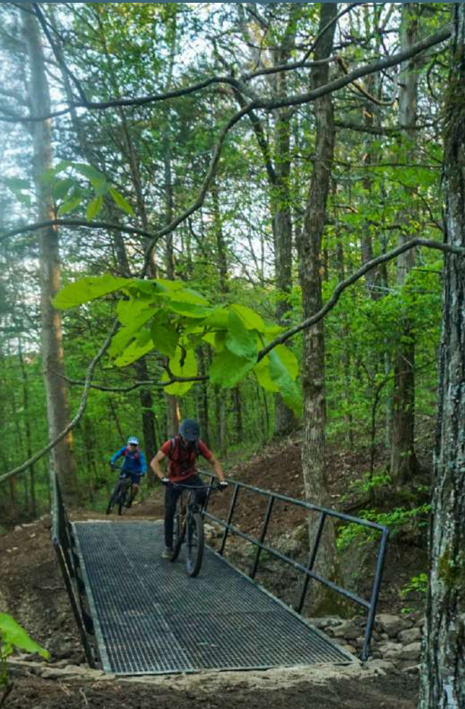
Prefabricated steel bridge at Devil's Den State Park in Winslow, Arkansas. Photo by Andy Flietstra/Rock Solid
