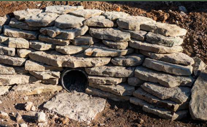
Small retaining wall with culvert. Photo by Eli Glesmann/Rock Solid
