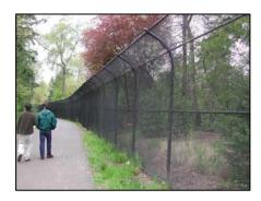
The high curved fences are typically a minimum of 12 feet in height and curved at the tops. The photograph above shows an example where the fence is painted black to blend with the landscape. Below, is an example of utilizing trees as a form of visual as well as protective screening for trail users. In many cases no fencing is needed due to golf course configuration and thorough understanding of possible golf ball trajectories.
