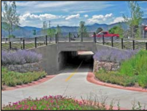
Cast-In-Place Concrete
