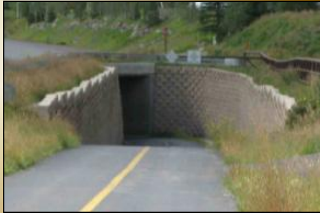
Mechanically Stabilized Earth
