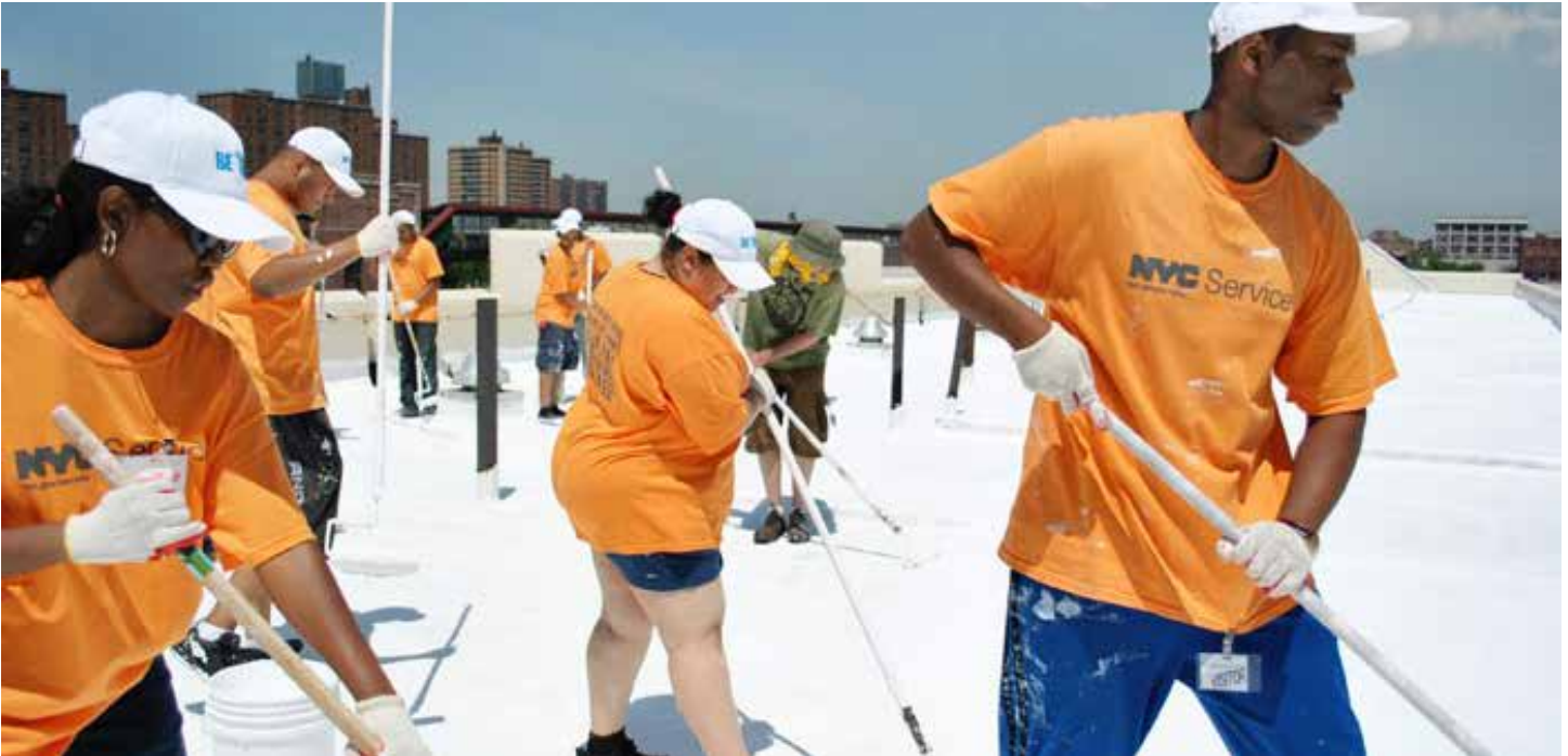
Corpsmembers painting a cool roof in New York City
