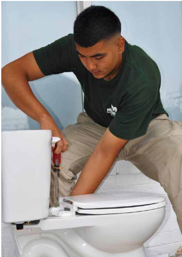
Corpsmember installing a water-saving toilet in a low-income home in Colorado
