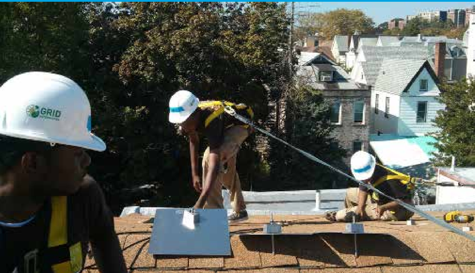
Corpsmembers installing solar panels in New York City
