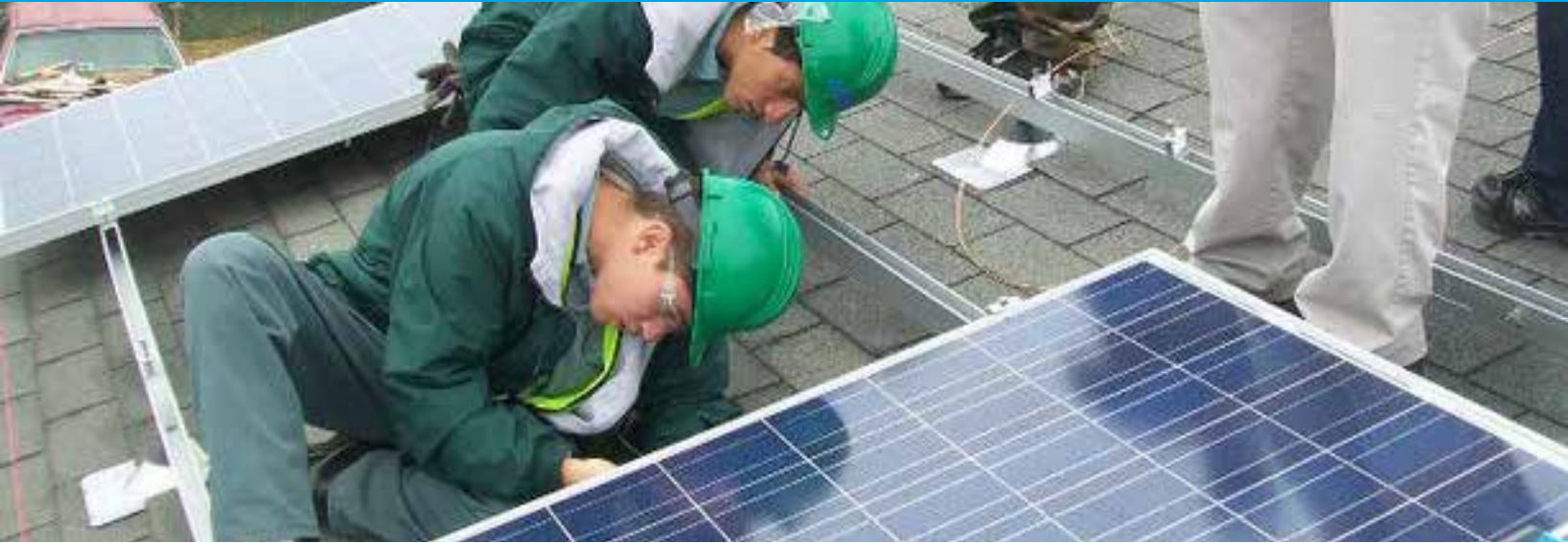
Corpsmembers installing a solar panel in Los Angeles, CA
