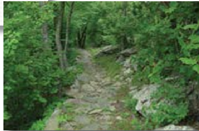
This section of the Appalachian Trail in Shenandoah National Park is improved by stone paving.
