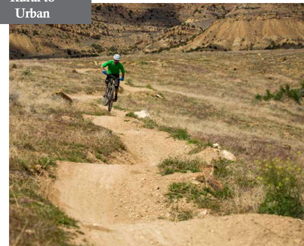
PBR Trail: Small/gentle rollers and berms, shape supported with rock materials, lots of undulations and meanders, flow adjusted to reduce speeds (to reduce breaking, sliding), soil amendments for tread shaping
