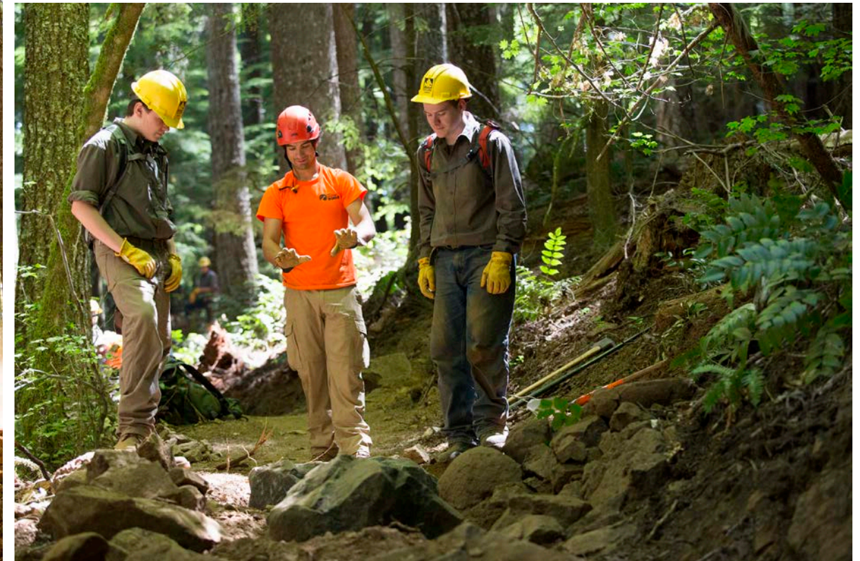
Whistle Punk construction specifications reflect the conceptual plan and design guidelines to produce the desired experiences. In this case, rock was imported and placed to provide more technical challenge than native materials could provide.
