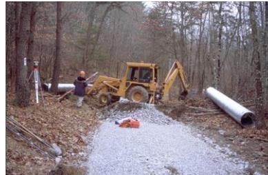
Figure 5. From top to bottom: typical examples of trail clearing, establishment of road surface, stabilizing the surface, installation of water control/stream crossing structures, and surfacing.
