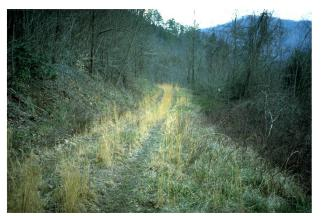
Figure 4. View of one road evaluated by Swift (1984) after the road has been stabilized with gravel and vegetation.
