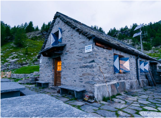
Oldest purpose-built mountain hut in world. Grunhorn 1863
